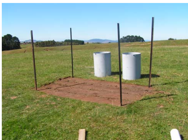
Figure 6.5 Recharge site prior to driving casings.
