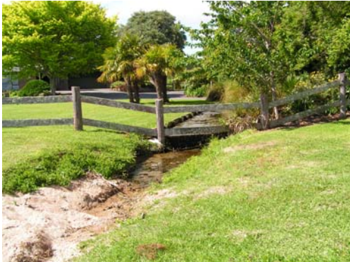
Figure 36.1. Drain with no water flowing, eastern Lake Rotorua.
