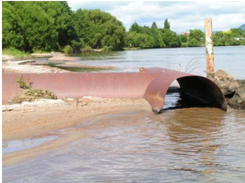
Figure 33.1. Large steel pipes have flowing water, eastern side of Lake Rotorua.
