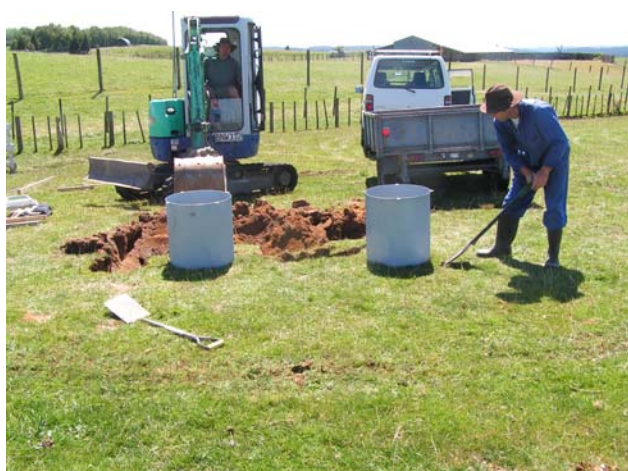
Figure 6.6 Initial placing of casing.
