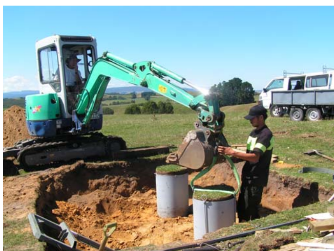
Figure 6.9 Lifting the soil column.
