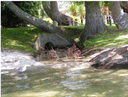
Figure 59.1. Water does not reach lake edge due to sandbank, near Rotorua's waterfront.
