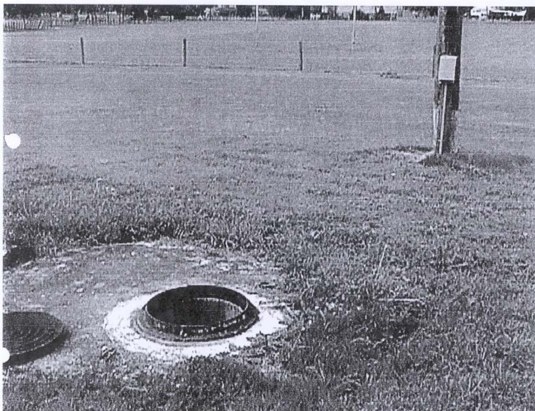
Existing (Production Bore 1) RDC Bore 4. Mamaku. Taonship.
