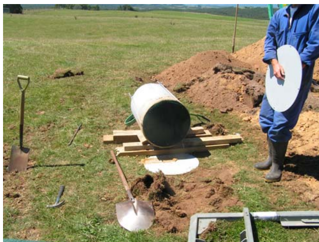
Figure 6.11 Base preparation of the soil column.
