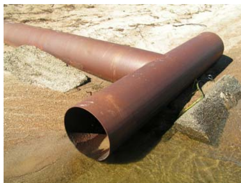
Figure 32.1. Steel pipes emit flowing water, eastern side of Lake Rotorua.
