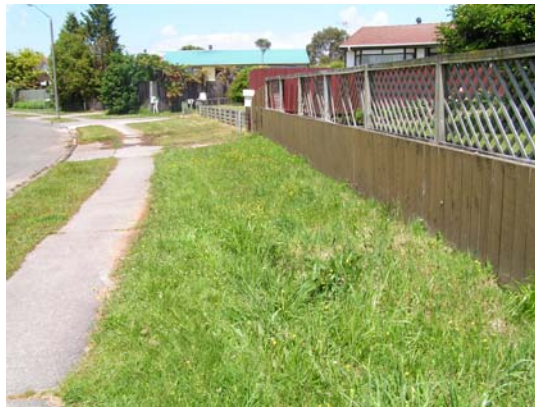
Figure 5.1. Seep in front of 48 Pohutukawa Drive, Rotorua.
