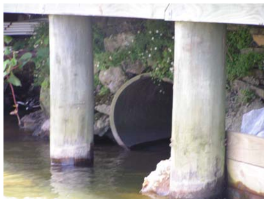
Figure 60.1. Large pipe at Rotorua's waterfront.
