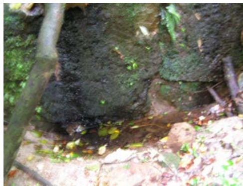
Figure 14.1. Seep emerging from bank, Mission Bay, Rotorua.
