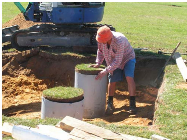
Figure 6.7 Casing excavation.
