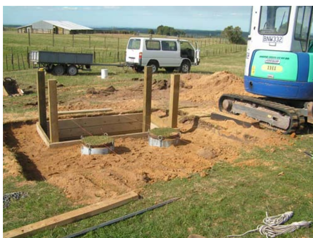
Figure 6.15 Backfilling the pit.
