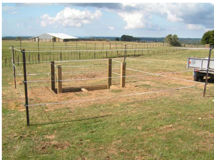
Figure 6.16 Completed lysimeter installation.
