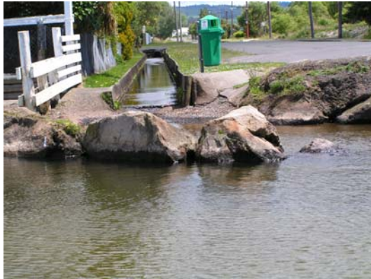
Figure 69.1. Eastern side of the road, water drains into Lake Rotorua.
