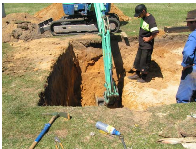
Figure 6.12 Digging the box section.
