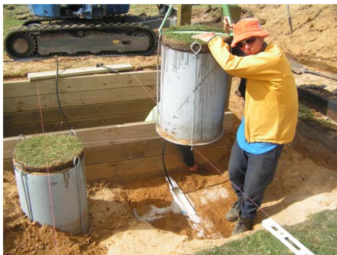
Figure 6.13 Lysimeter installation.
