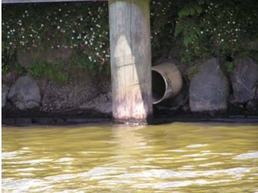
Figure 60.2. Drainage pipe at Rotorua Lakefront.
