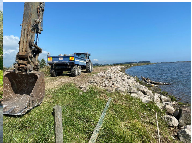
Maketu Foreshore stopbank armour
