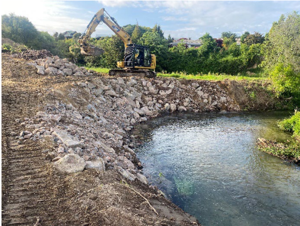
Utuhina stream rock erosion repairs
