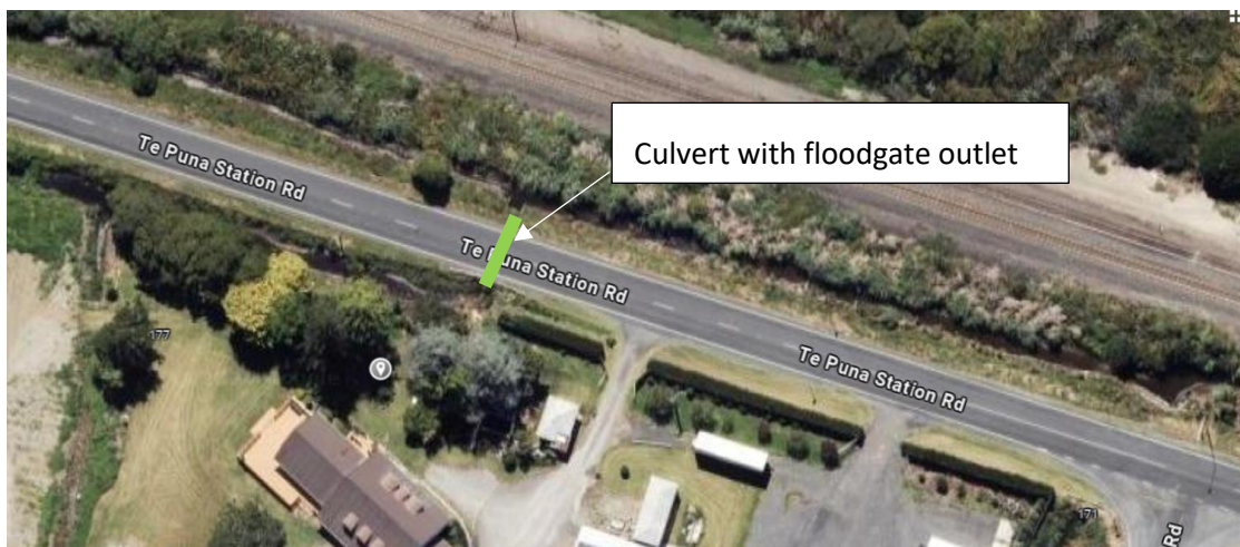
Figure 5: Location of culvert under Te Puna Station Road
