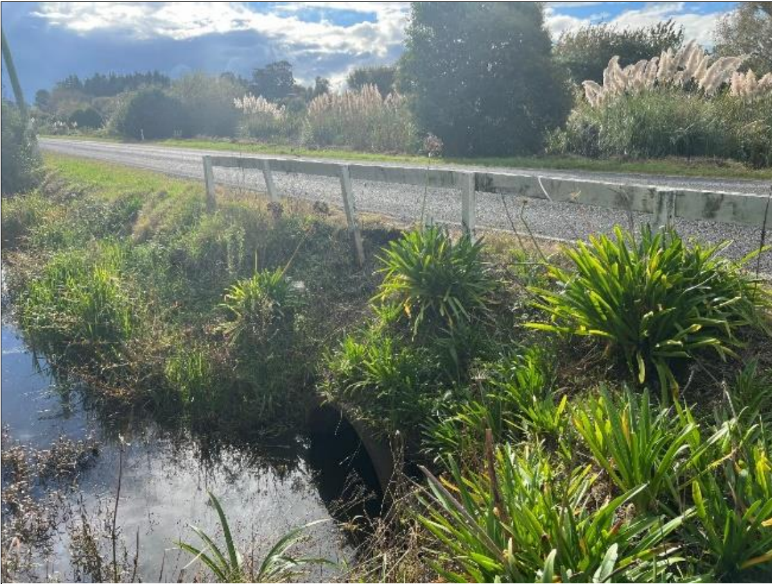
Figure 6: Inlet of culvert under Te Puna Station Road
