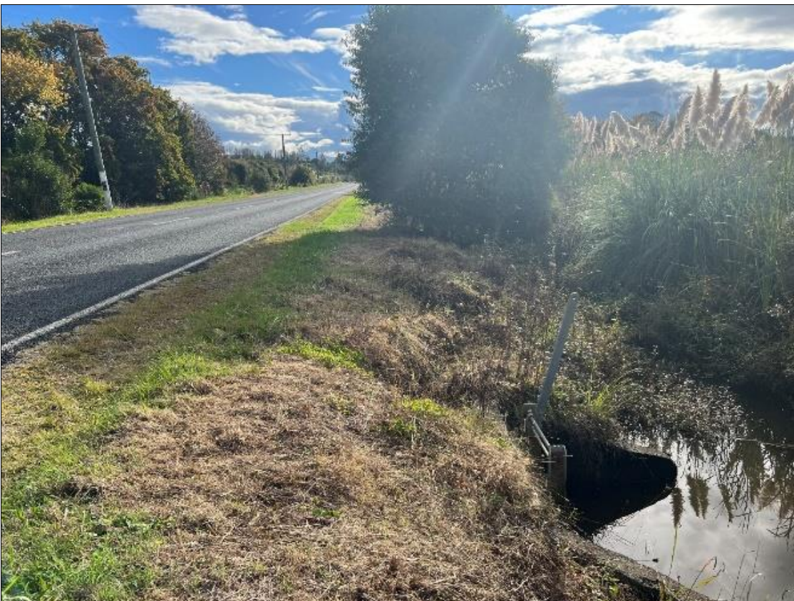
Figure 7: Floodgate on outlet.
