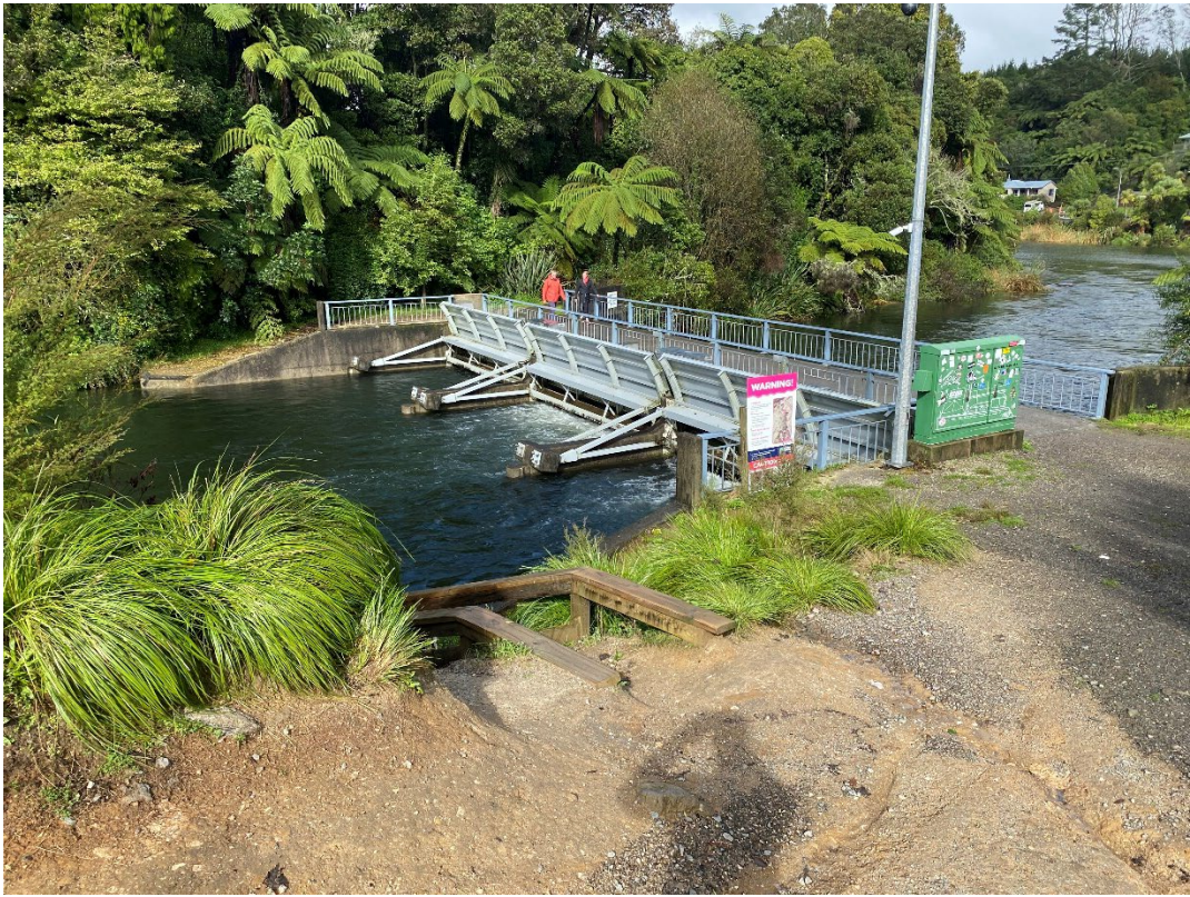
Figure 15 Okere Gates fully open - Lake Rotoiti at 279.425 m 10 May 2023
