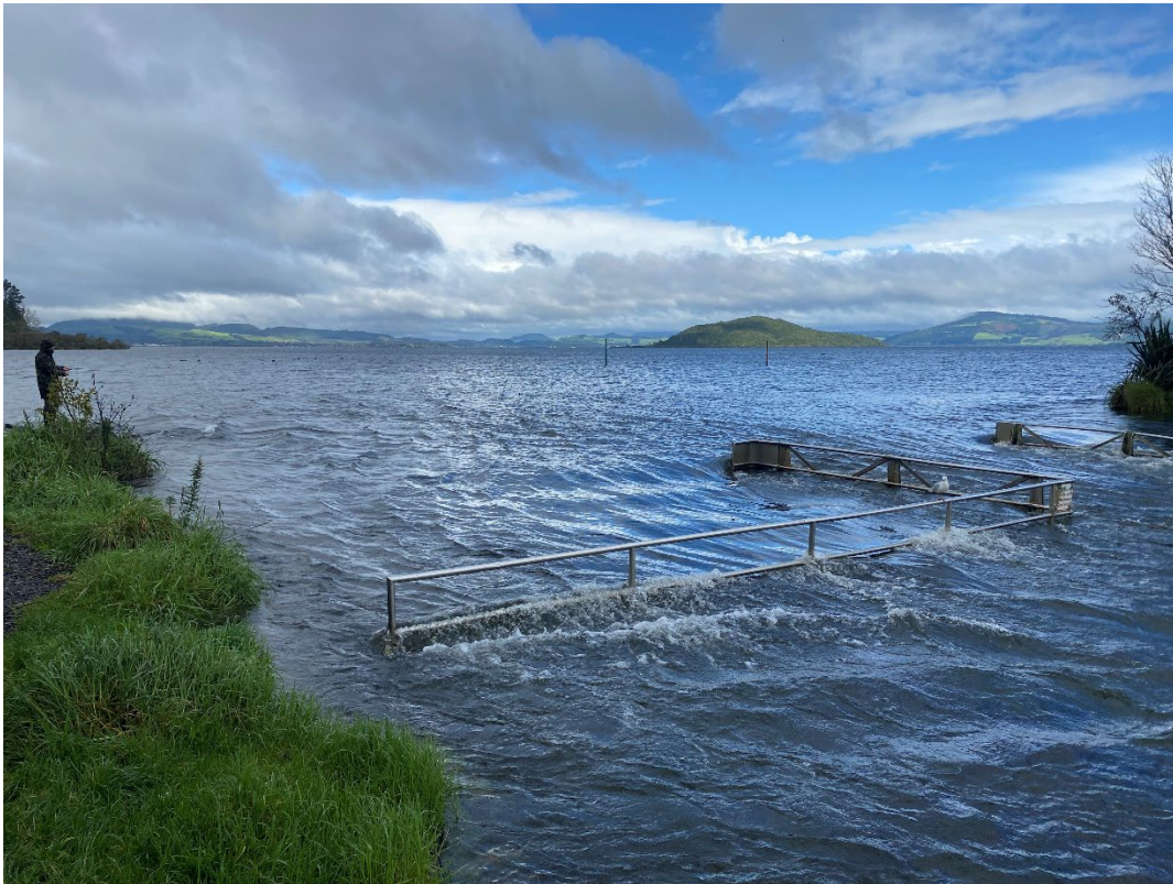
Figure 3 Ōhau Weir Lake Rotorua - Lake Level 280.295 m 10 May 2023
