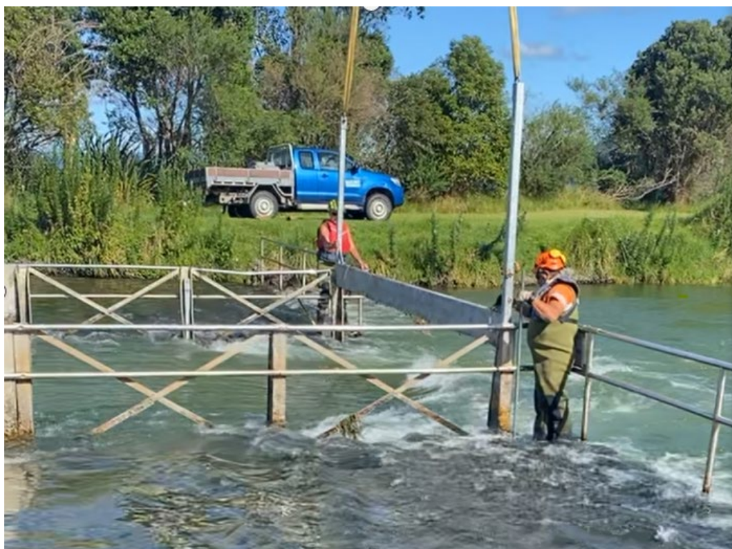
Figure 16 Installing the Ōhau Channel stoplogs 29 February 2024
