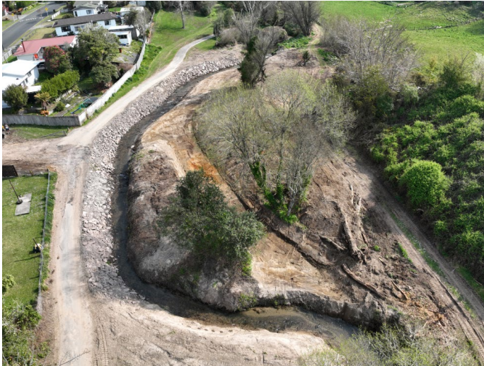
Mangakakahi Stream floodway clearing
