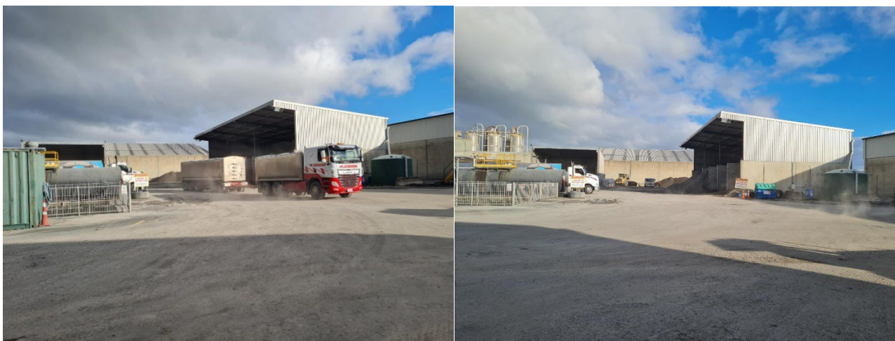
Figures – Aggregate storage sheds on western boundary of site. Dust visible.
