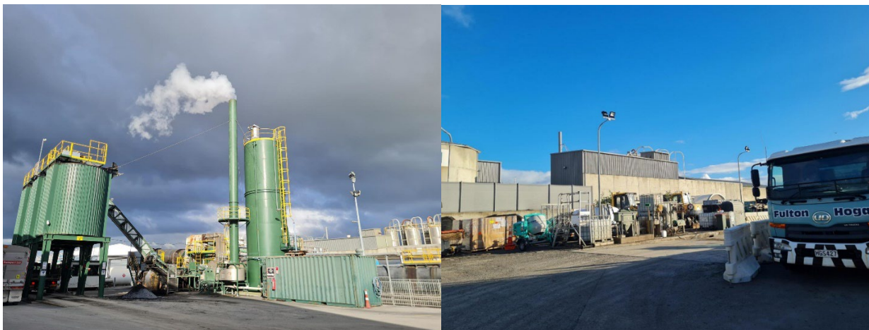
Figures - Existing plant (left) and storage area behind office, southern boundary of the site (right).
