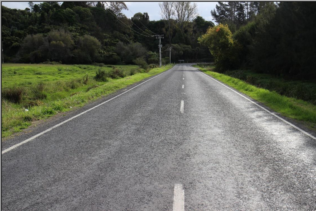
Photograph 3: Te Puna Station Road Looking West
