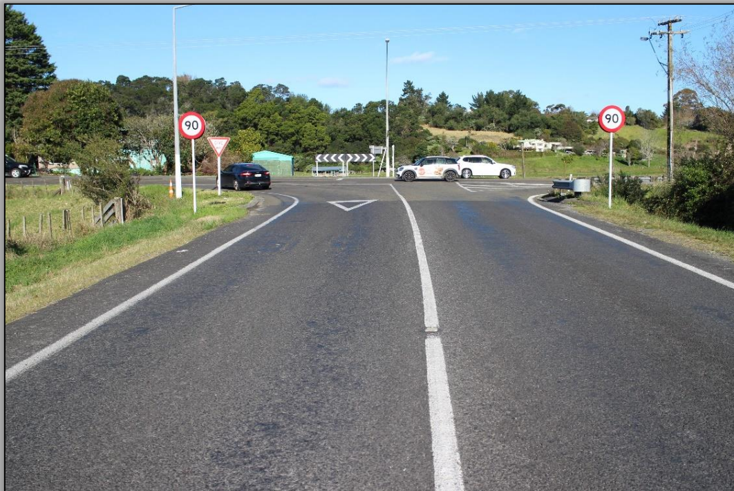
Photograph 4: Te Puna Station Road Approach to SH2
