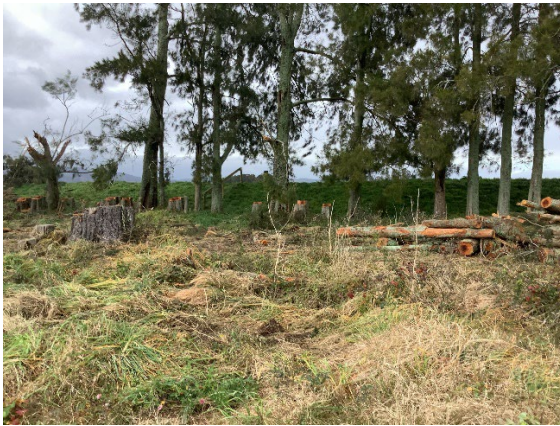
Rangitāiki stopbank asset defect repair
