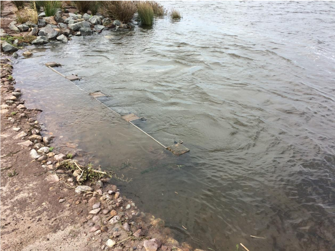
Photo 21: Te Pa Ika culverts outlet
