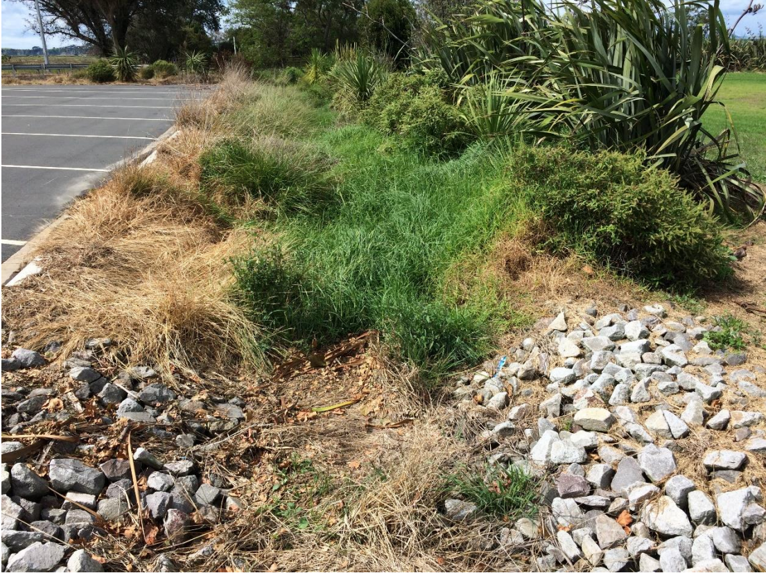
Photo 11: Car park swale drain
