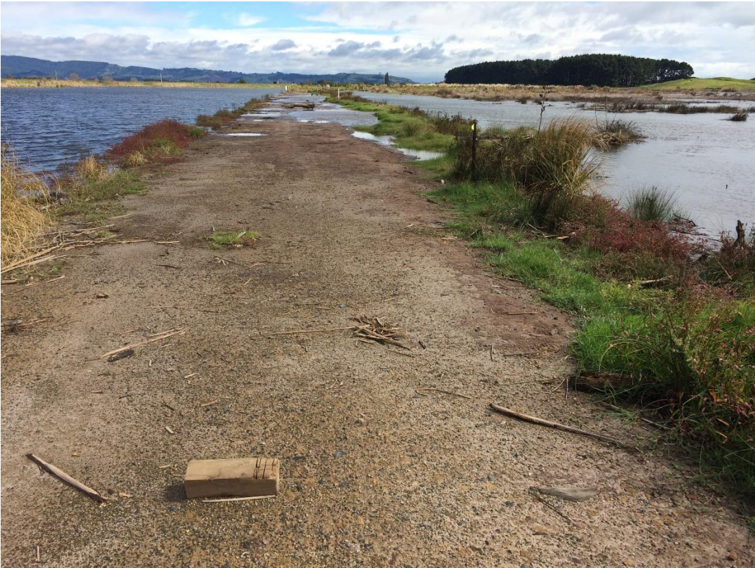
Photo 7: Left bank bund along new channel
