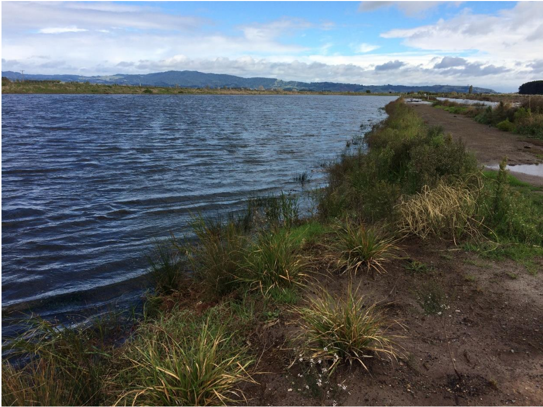
Photo 8: Left bank bund along new channel from outlet
