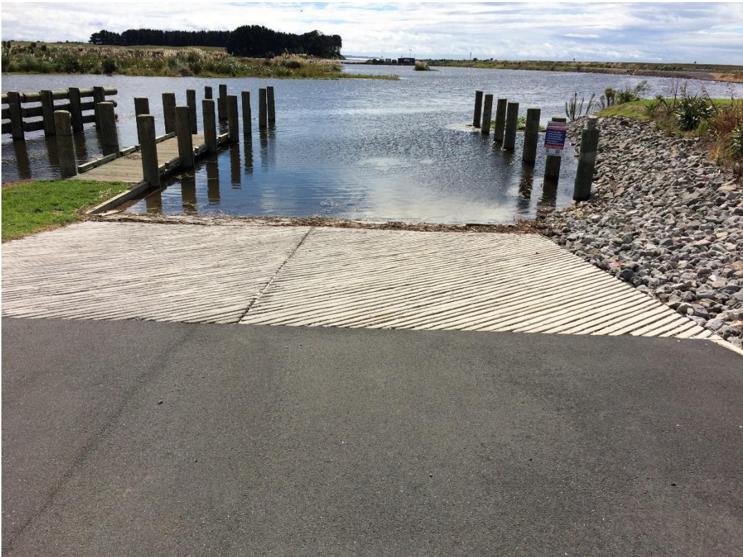
Photo 10: Boat ramp and public jetty
