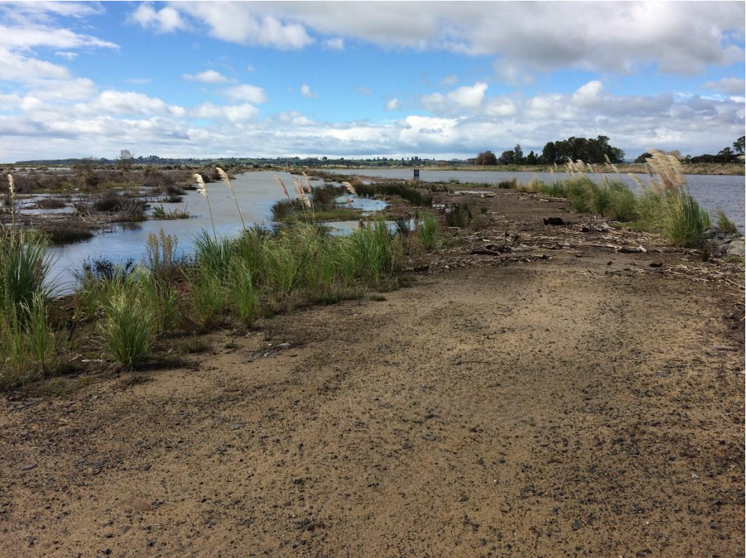
Photo 6: Left bank bund along new channel
