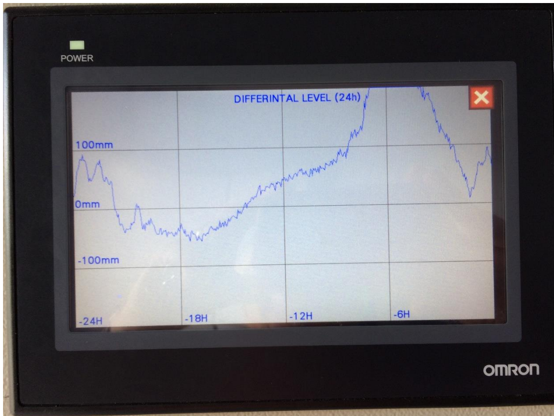
Photo 1: Differential water level across gates over the previous day (the gates may have been open for over 12 hours)
