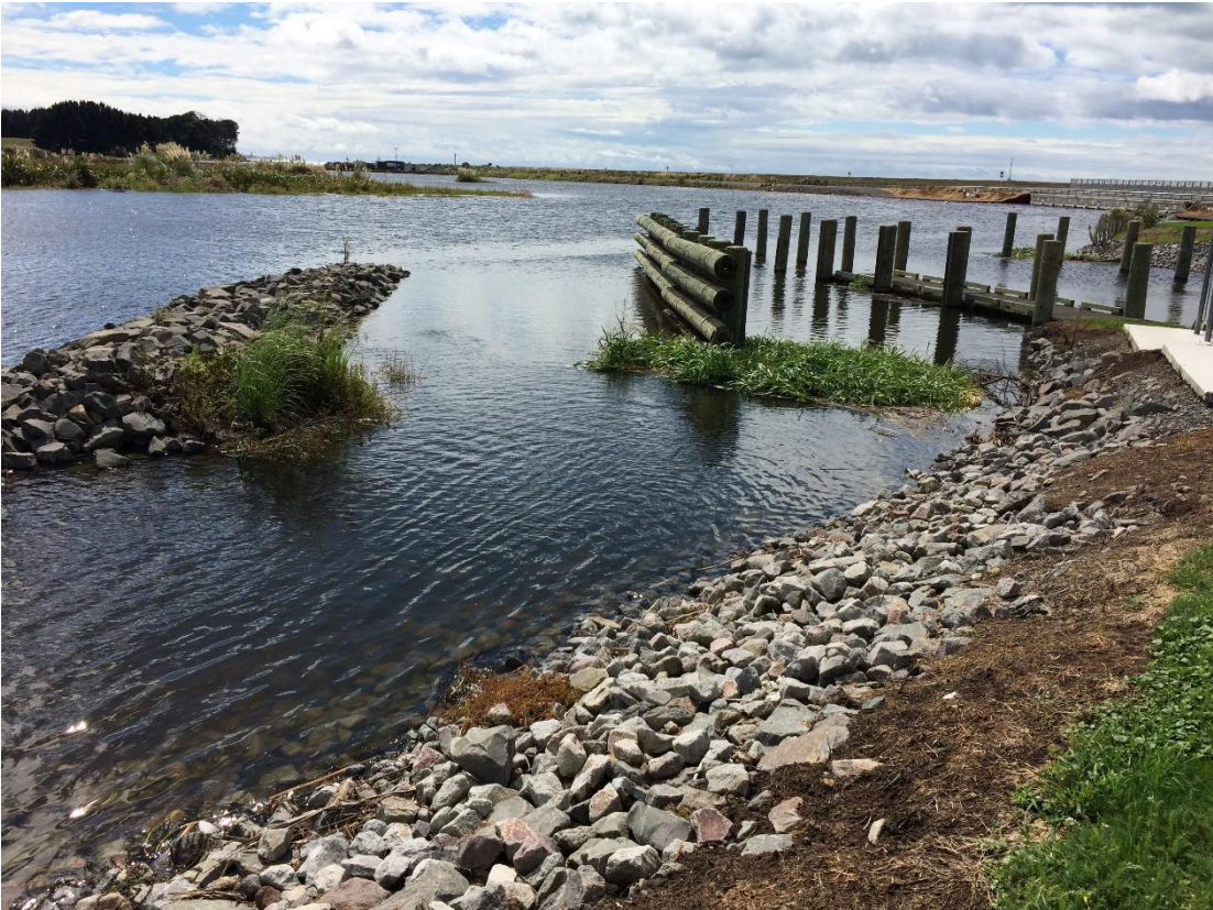
Photo 9: Rock bund and log deflector
