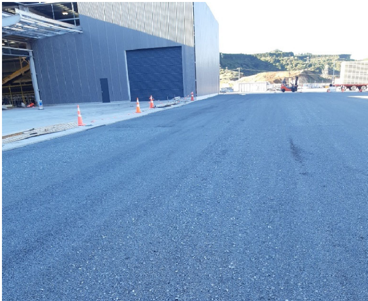
GIB facility – yard car park
