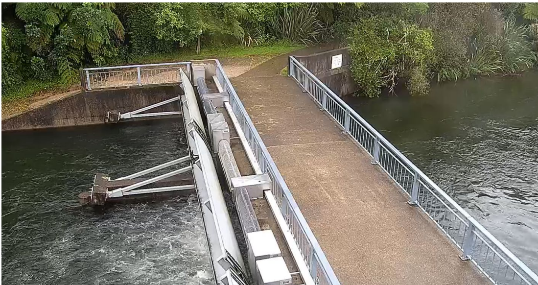
Figure 17 Okere Gates structure fully open to relieve lake levels above consented maximum February 2023
