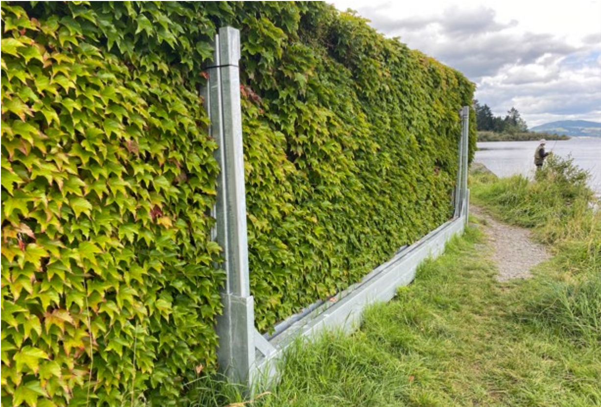
Figure 1 Ōhau Weir stoplogs – ready for BOPRC Rivers and Drainage staff and contractors to reinstall when lake levels are lower - 26 January 2023
