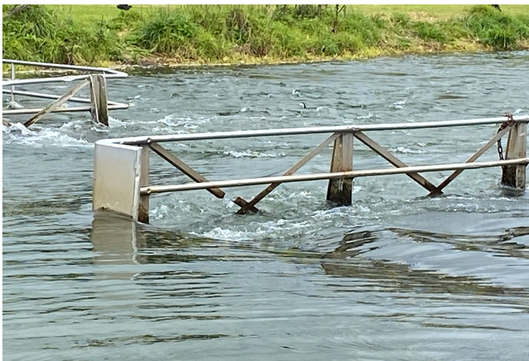
Figure 18 Ōhau Weir maintenance
