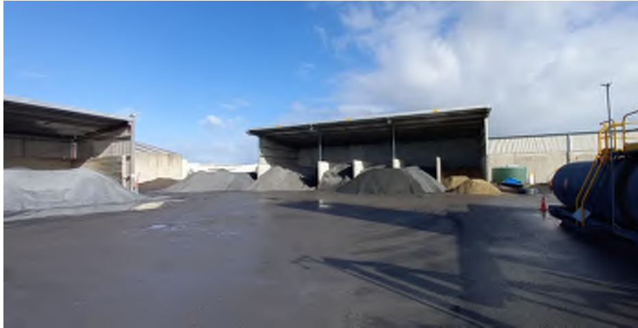
Photo 1: Aggregate Bay storage sheds one located in the middle of the south end of the site (left) and the other located along the western site boundary (centre).
