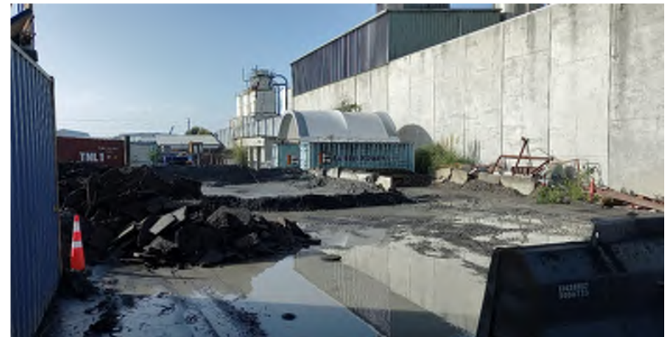
Photo 8: South-eastern corner of the site containing a drying area for sediments from the overflow pond (centre of image) and maintenance area storing tools (the far right) against the southern site boundary.
