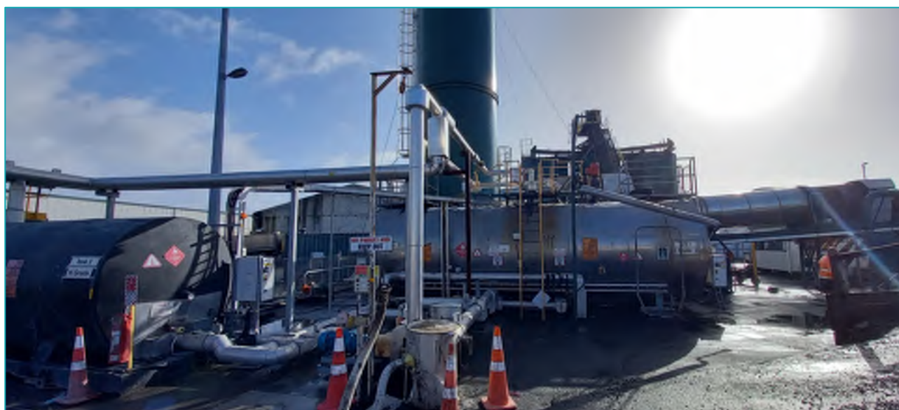
Figure 3. Photo of current asphalt plant (Beca photo 2.6.22)
