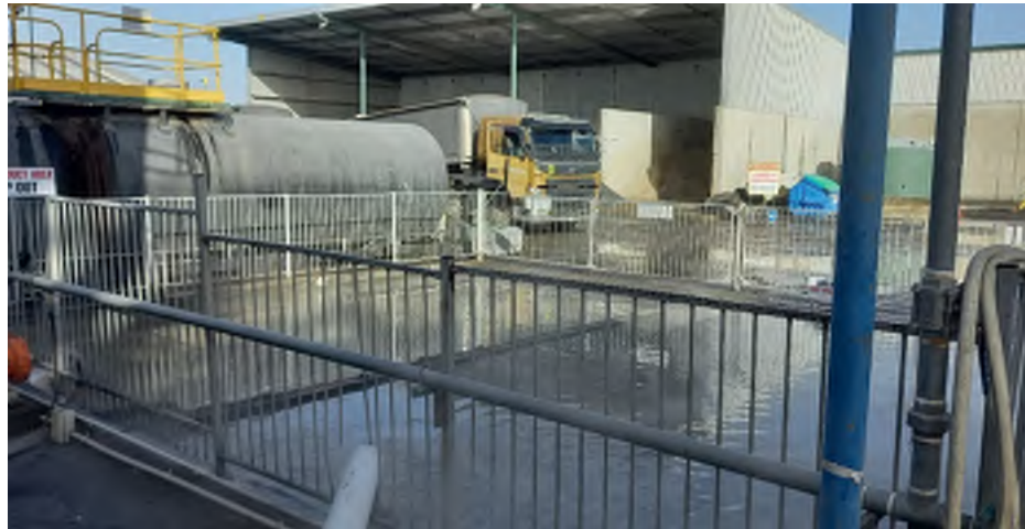
Photo 15: Water retention ponds located directly to the west of the asphalt plant and directly north of the black bitumen tank.
