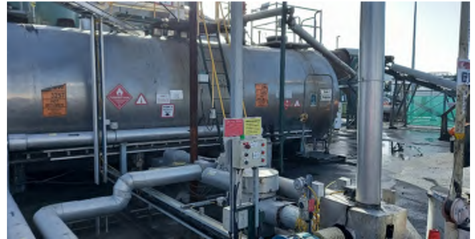
Photo 4: Hot Bitumen tank located directly to the east of the silo.
