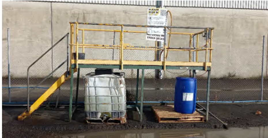
Photo 13: Truck wash station with white water tank and blue 400 Litre container of Bitumen release product. This is located outside the site.
