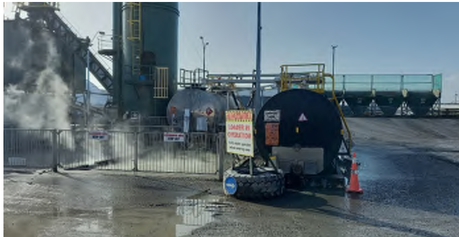
Photo 11: Overview of the asphalt plant looking towards the east. Asphalt plant including retention ponds, bitumen tanks, and lime silo in the foreground and portable hot storage hoppers in the background.
