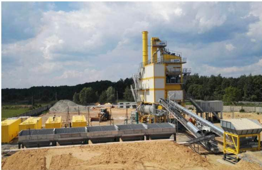
Figure 3.1: Marini 2500 batch mix plant
