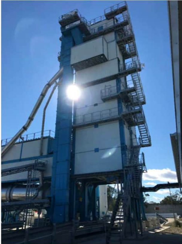
Figure 3.2: Marini Top Tower 3000 as installed in Sydney, Australia.
