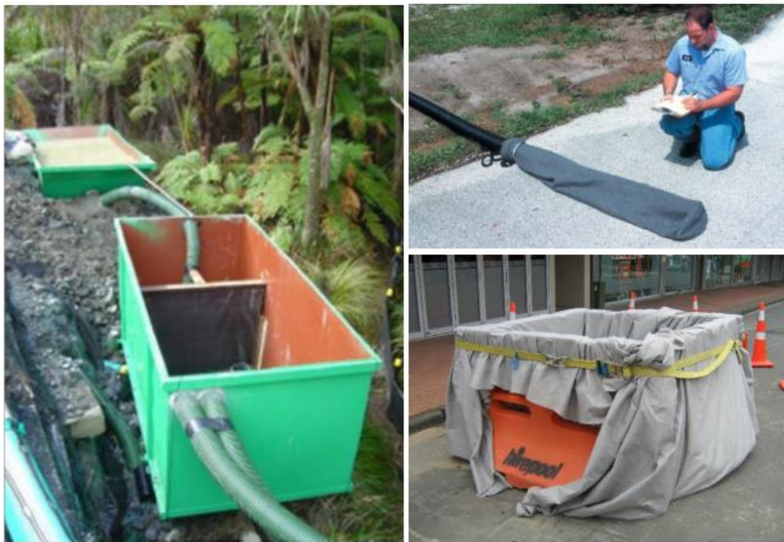
Figure 5. Example dewatering devices (source: Auckland Council Guideline Document 005)
