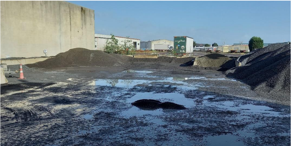
Figure 2. Aggregate stockpiles within the south-western corner of the site.
