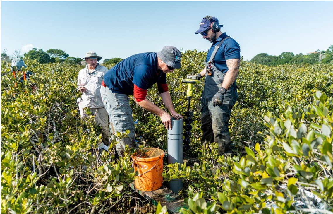
Figure 2-9: Battery powered post-hole borer used for installing hole for the PVC collar. A bucket and trowel is used to collect sediment removed from the hole for disposal away from the sample station.
