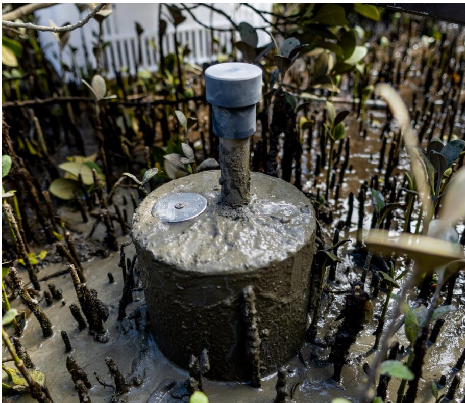
Figure 2-15: Completed RSET benchmark with stainless steel identification tag. The receiver is fixed to the RSET rod that is encased in concrete inside the PVC collar.
