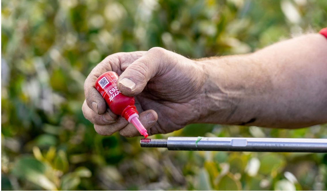
Figure 2-11: Thread locker applied to threads of SS rods.
