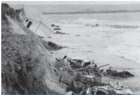
Ohiwa 1976 erosion. The buffer here was too narrow to cope with natural processes.
