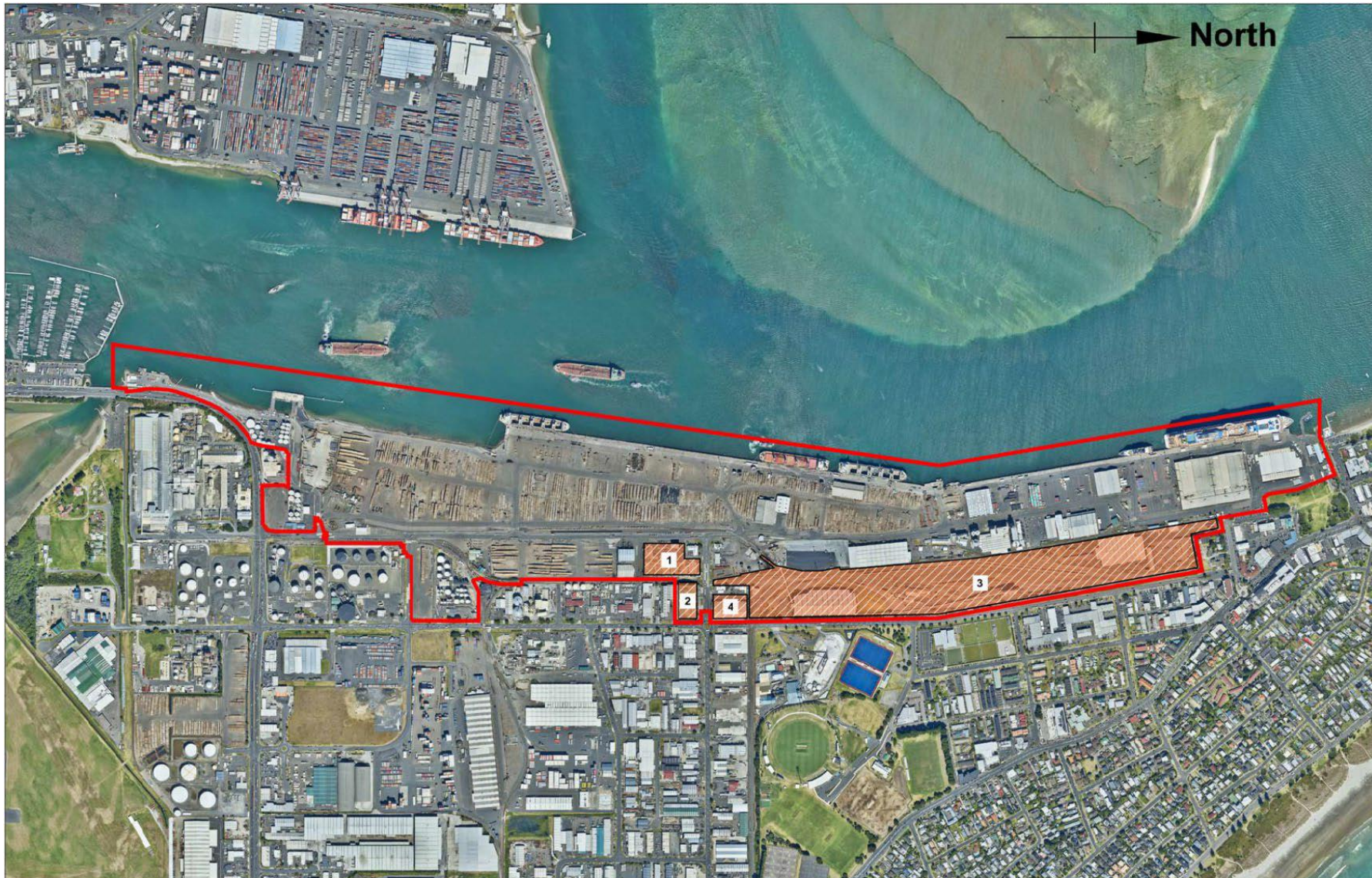
Figure 1: Aerial image showing the extent of the Port of Tauranga “subject site” for the purpose of the PC13 rules
