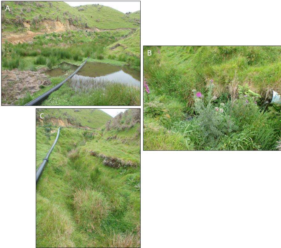
Figure 3-13: Site 4 in Onepu Stream in 2012. A, upper wetland; B, perched culvert at the base of the wetland; C, ephemeral stream below the wetland. Water pipes currently run adjacent to the stream and through the wetland.
