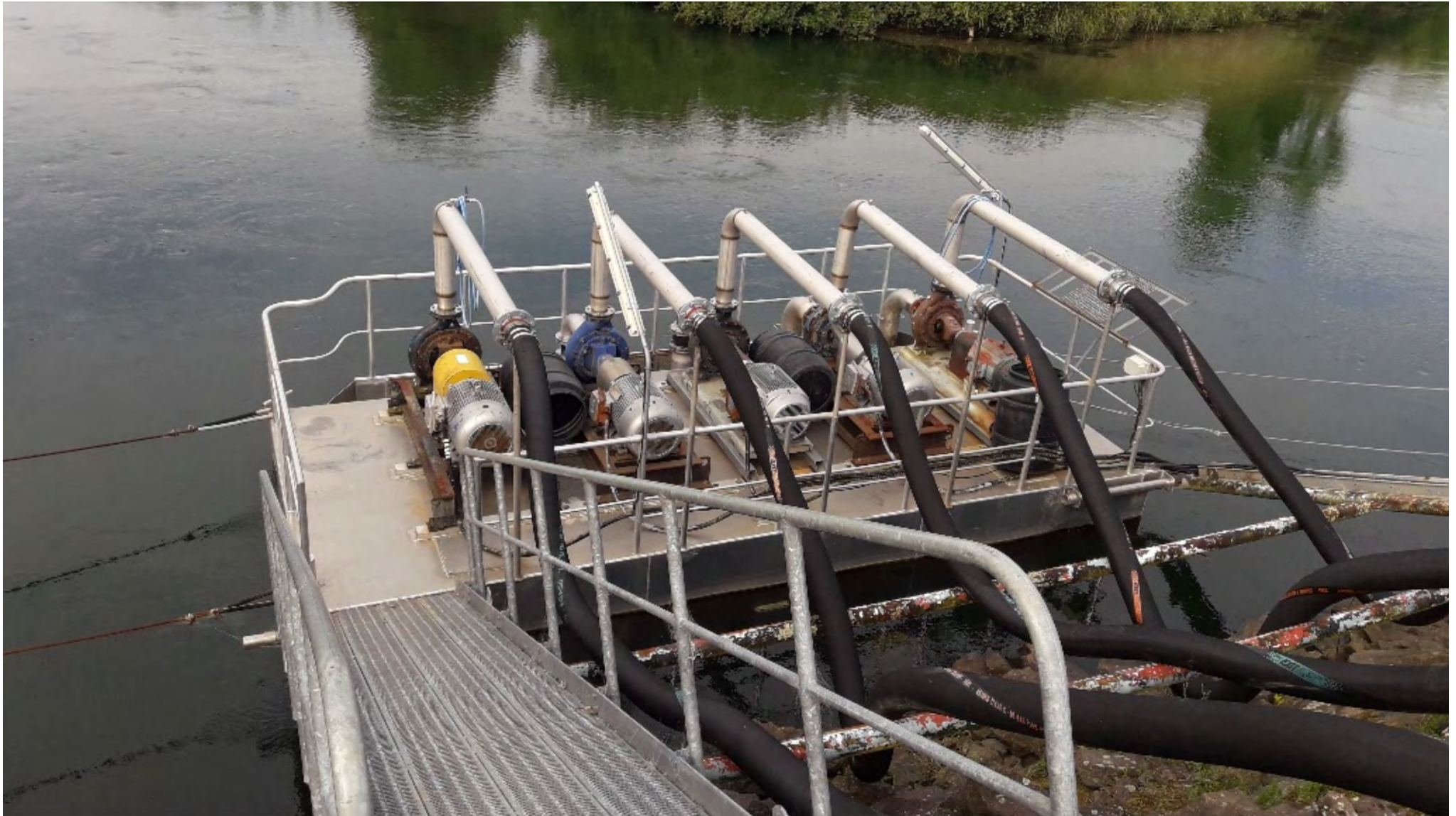
Figure D – Barge with Intake Pumps
