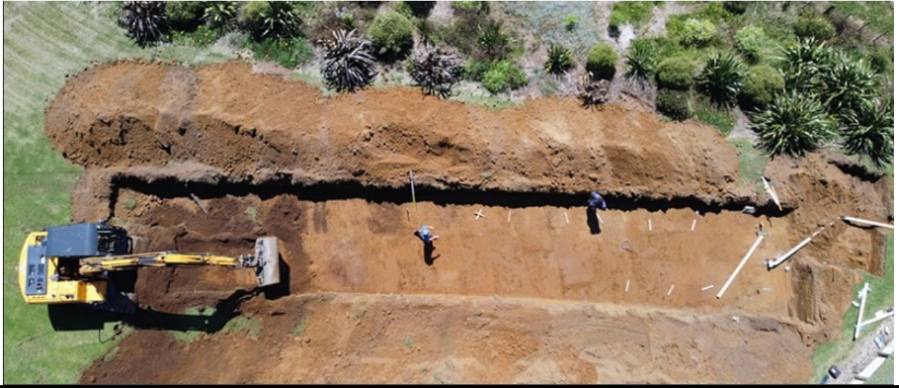
Figure 25 Foundation preparation for a new detention dam site
