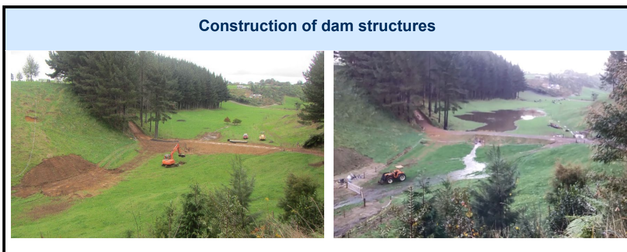
Figure 10 Construction of dam structures
