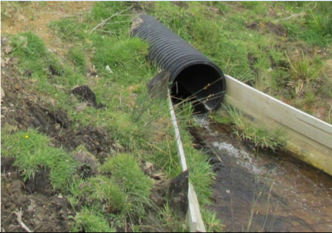
Figure 28 Example of a detention dam outlet with a timber discharge chute
