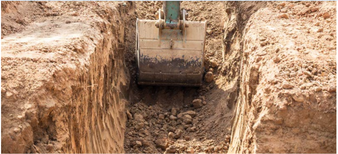
Figure 26 Excavation of a cut-off trench
