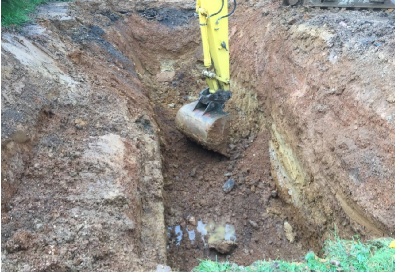
Figure 18 Photo showing excavation of weaker soil below a new detention dam
