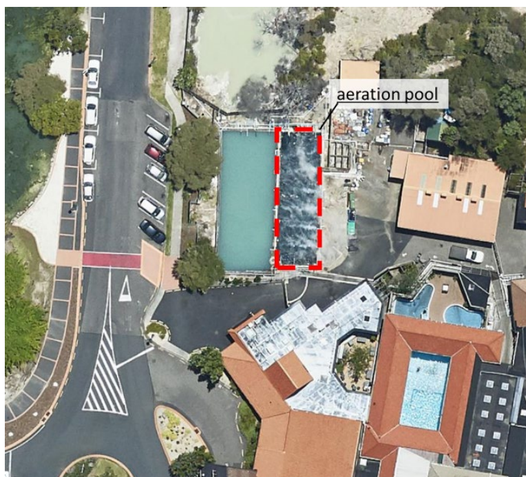
Figure 1.6 Example of an aeration pool (aeration tank) in Rotorua.
