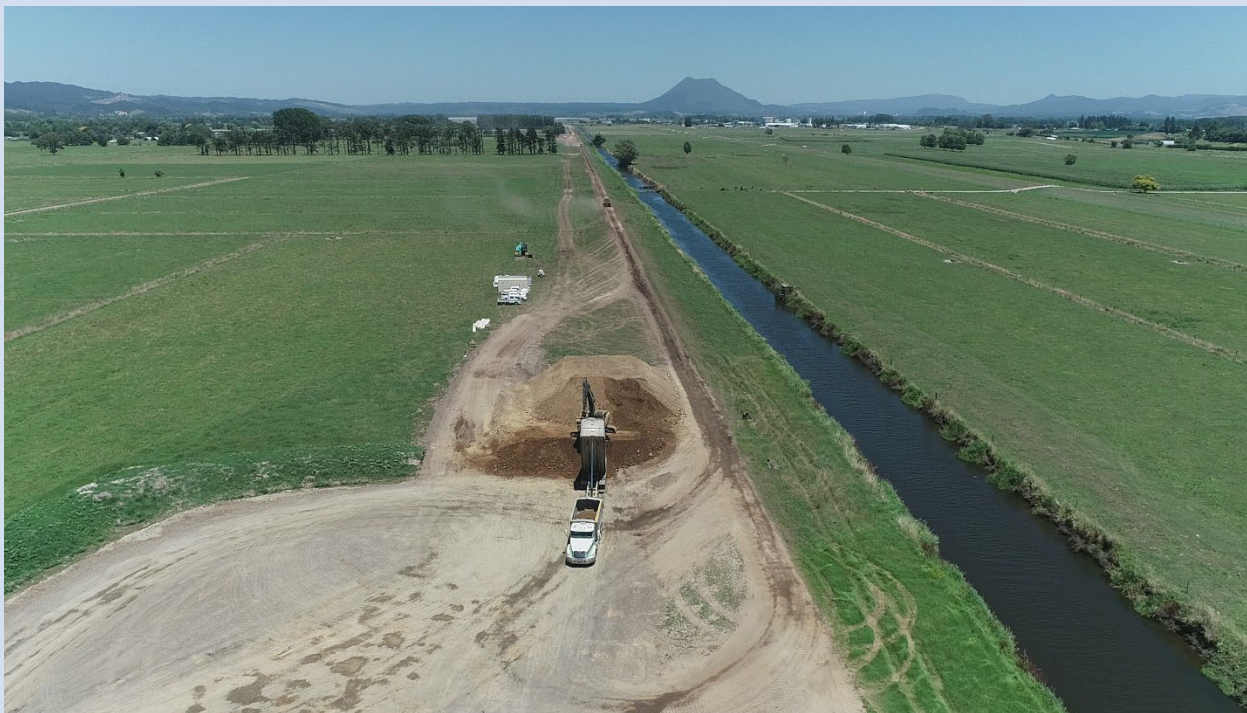
Stage 6C Earthworks
