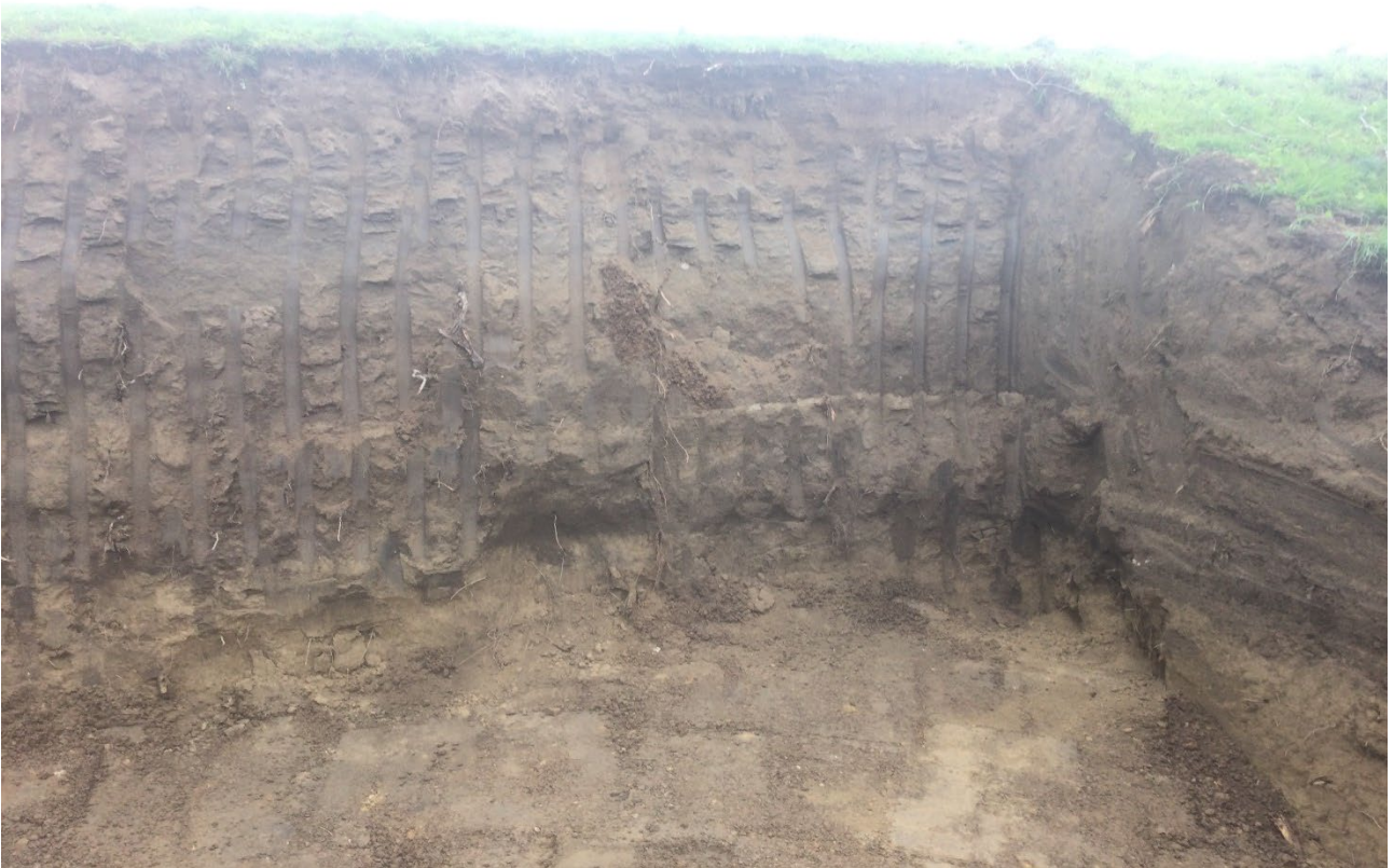
Tree roots excavated – extends to well into stopbank (above)
