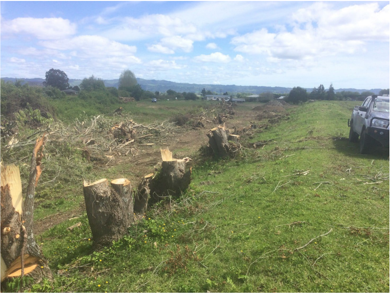
Trees along toe of stopbank (above)
