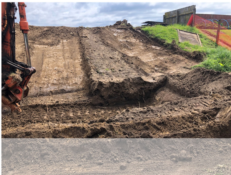
Photo 2 - Stopbank previously heavily planted and within a private fence line being remediated
