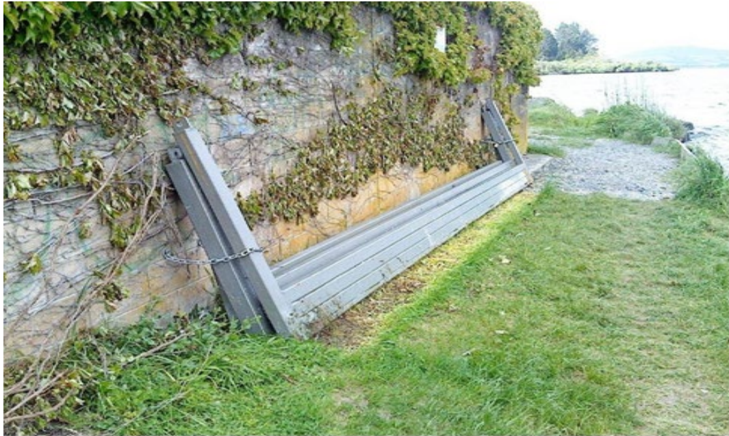
Figure 10 Ohau Channel stoplogs stored on site following refurbishment. Each stoplog (x3) is 6 m long x 0.3 m high.
