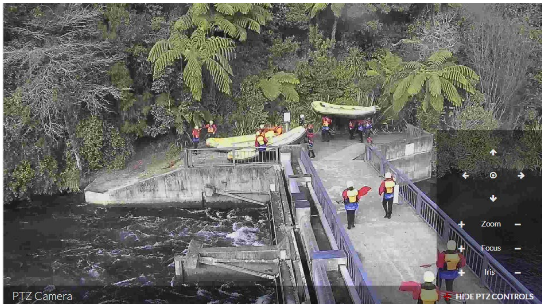
Figure 15 Rafters preparing to enter the Kaituna River from Okere Gates structure.
