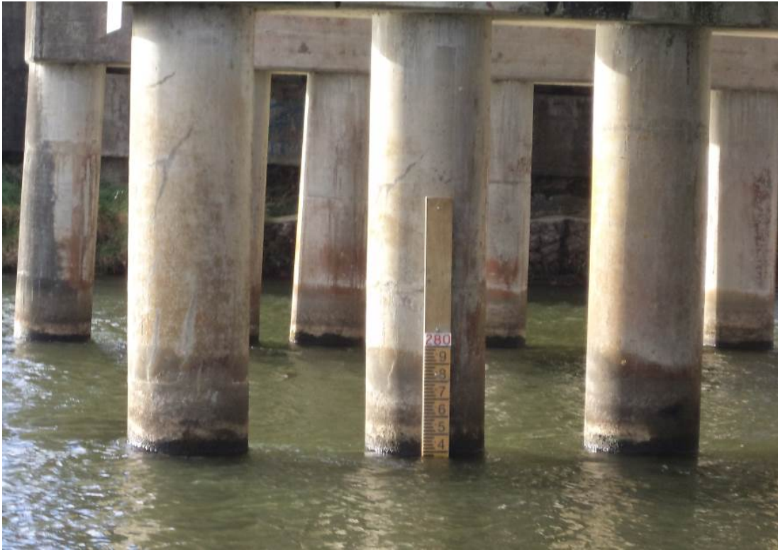
Figure 18 Ohau Channel Staff Gauge on State Highway 33 Bridge – Mourea.
