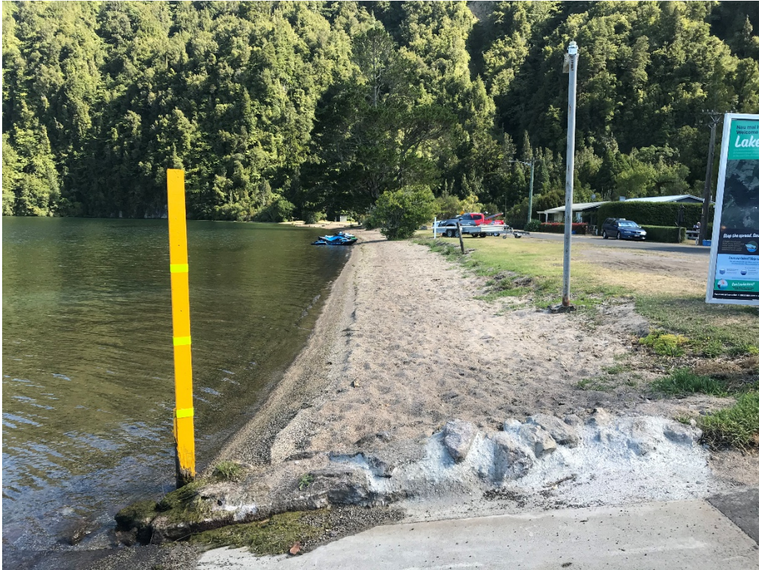
Figure 7 Lake Rotoiti at Hinehopu during summer – Lake Level RL 279.052 m – 2 February 2021.
