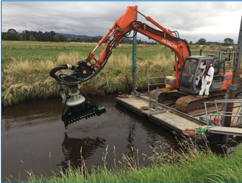
Photo 3: Sediment dredging in the canal in early January 2018.
