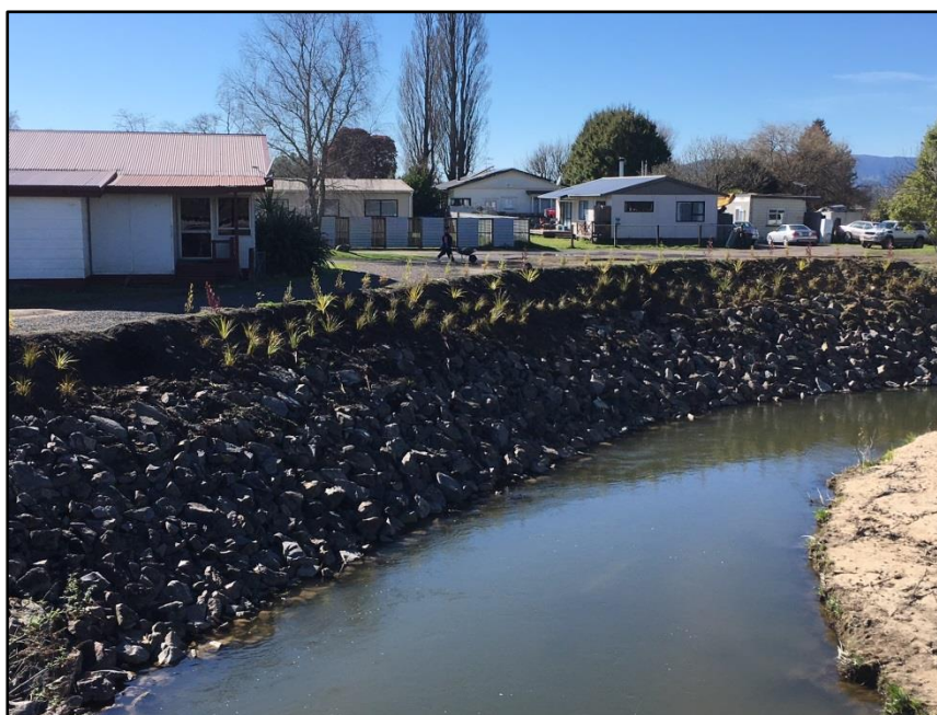
Photo 3 : Erosion repair work behind Parawai Marae.
