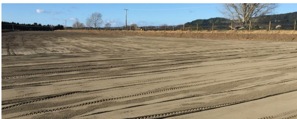
Figure 6. Containment Site 3 – construction complete and ready for lining.
