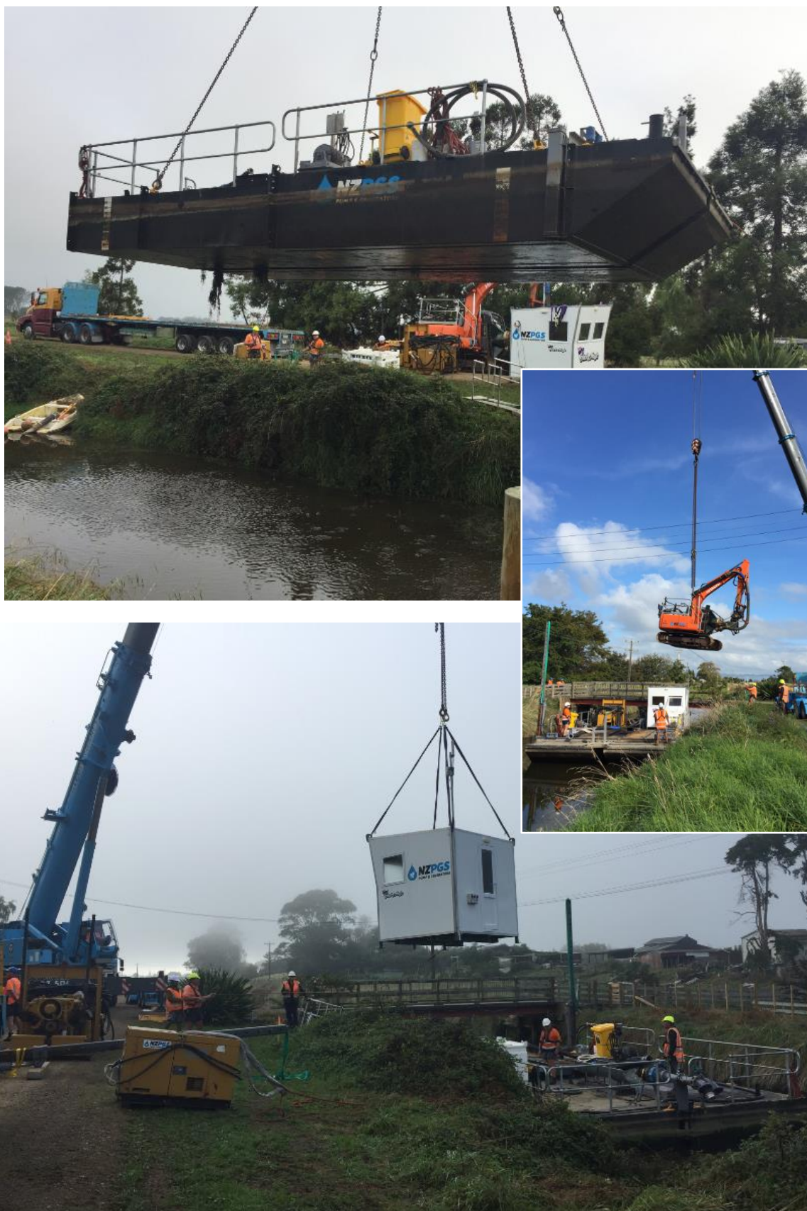
Figure 3. Barge and dredge lift over second private bridge.
