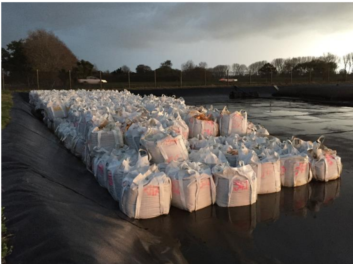
Figure 5. Oversize material (>4mm) in bulk bags within the Containment Site1 cell.
