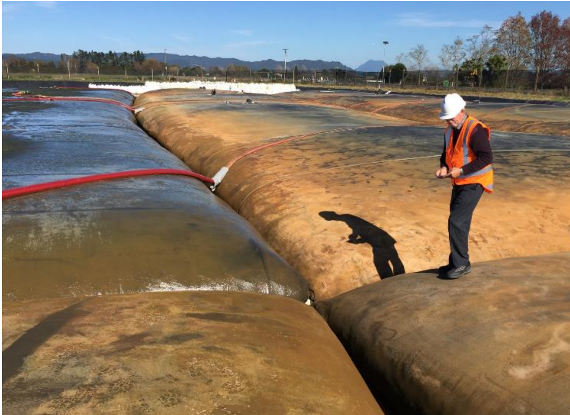
Figure 4. Geobags filled at Containment Site 1.
