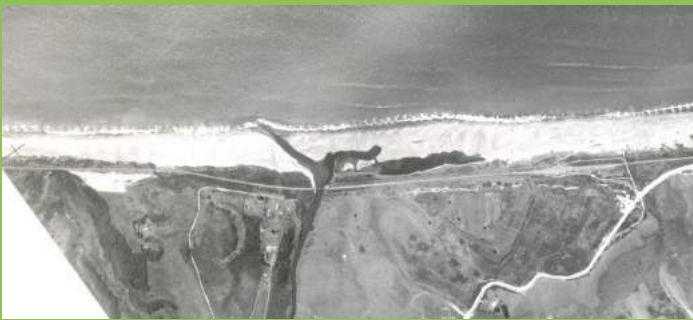
March 1943: Earliest photography showing confinement structure on right.
