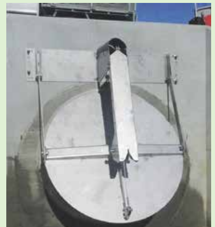
Fish friendly flap gate on the Ohau River, Levin.
