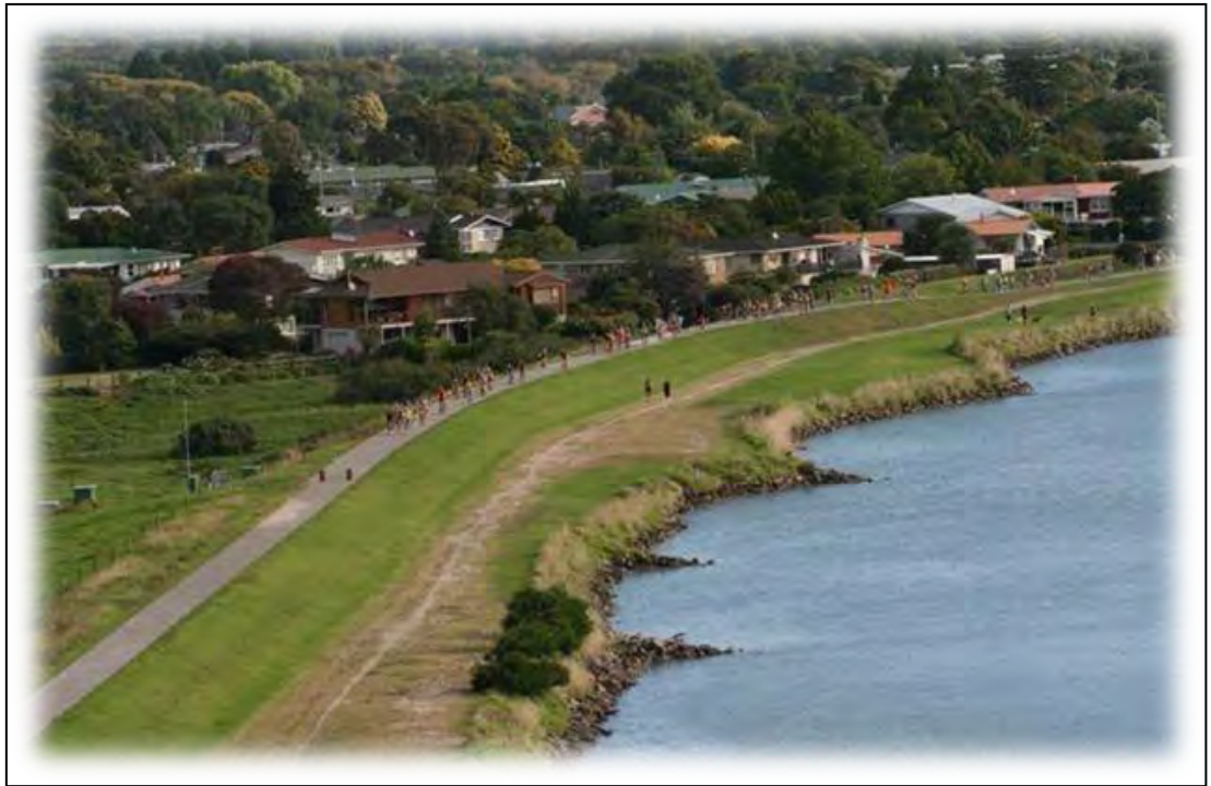
Figure 30 This cycleway in Whakatāne is built on the river stopbank which also protects the town from flooding.
