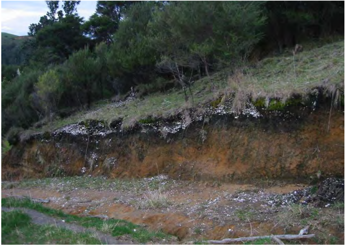
Figure 17 Midden eroding from face of cutting for a farm track.
