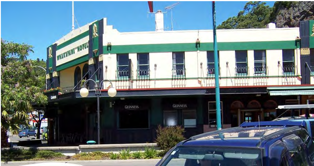
Figure 20 Whakatāne Hotel is an example of an Art Deco building.
