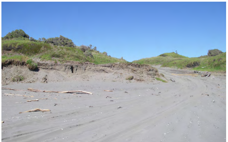
Hikuwai Beach - well-used vehicle access track and eroded fore dune
