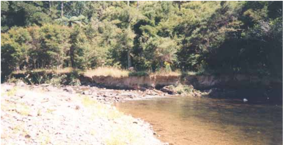
Figure 24.3 Erosion of the true left bank.
