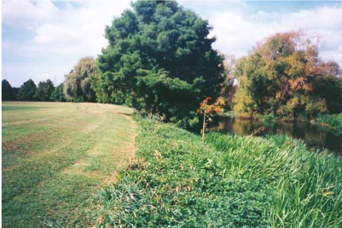
Figure 6.7 Stopbanking around the playing fields appears to be in excellent condition. Here, the stream is very wide (35m at the footbridge by the grounds) and slow-flowing.
