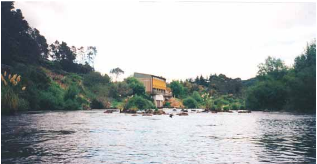
Figure 8.3 Shallow rocky bed at the Ruahihi power house.
