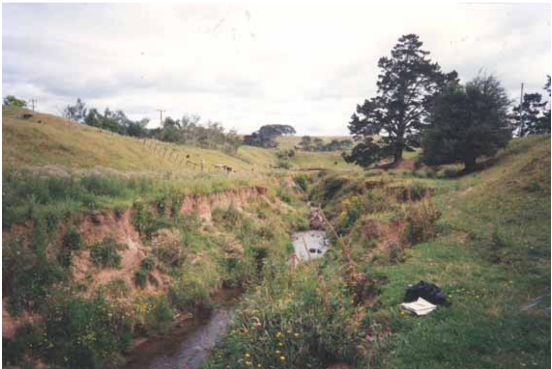
Figure 20.4 Erosion of the 2m high banks at 3.2km.
