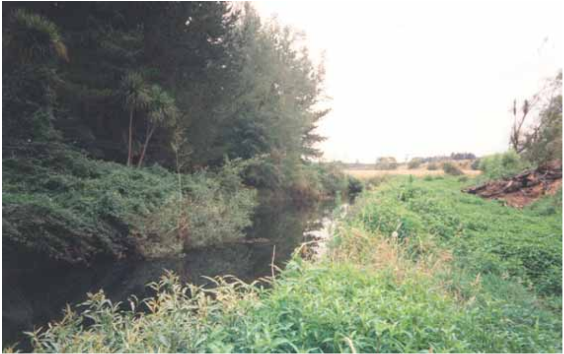
Figure 17.8 Banks become well vegetated with little erosion. Stockpiled cleared vegetation have been burnt (seen to the right of the stream) often exposing the stopbank.
