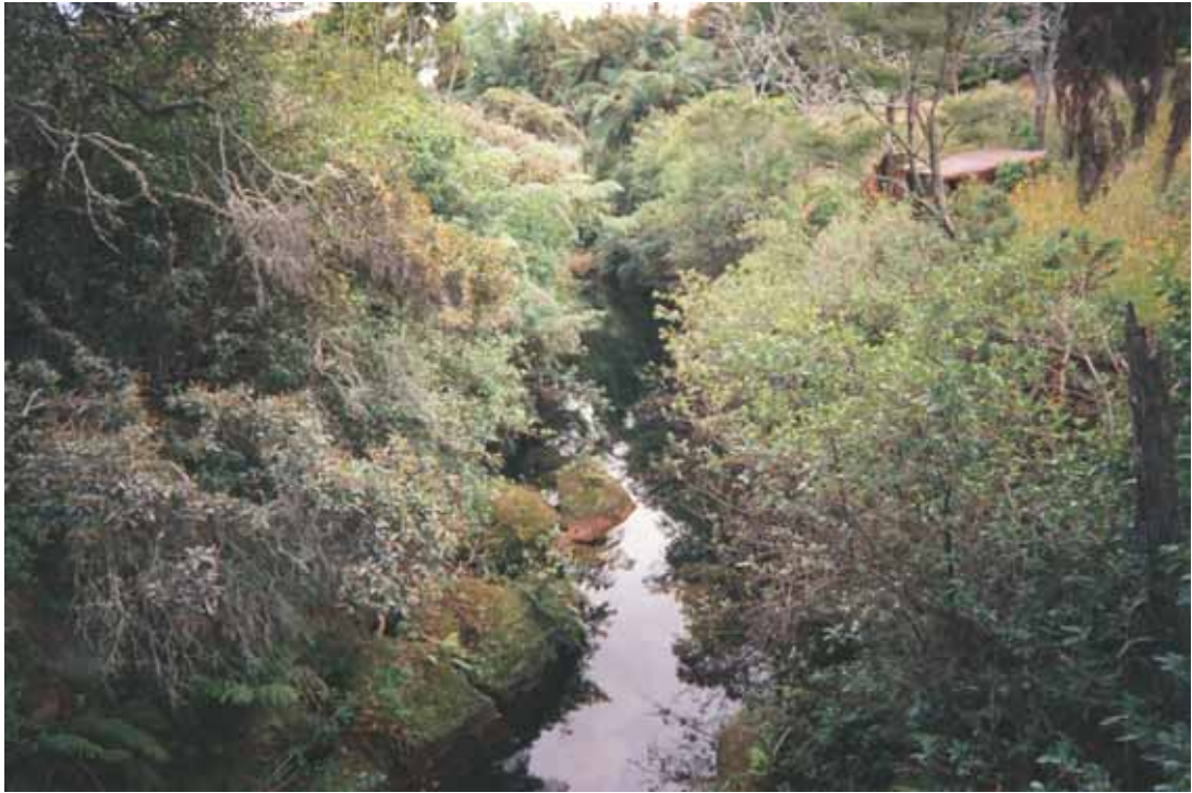
Figure 15.1 Looking downstream from Upland Road bridge. Banks have a thick vegetation cover, and erosion is minimal.
