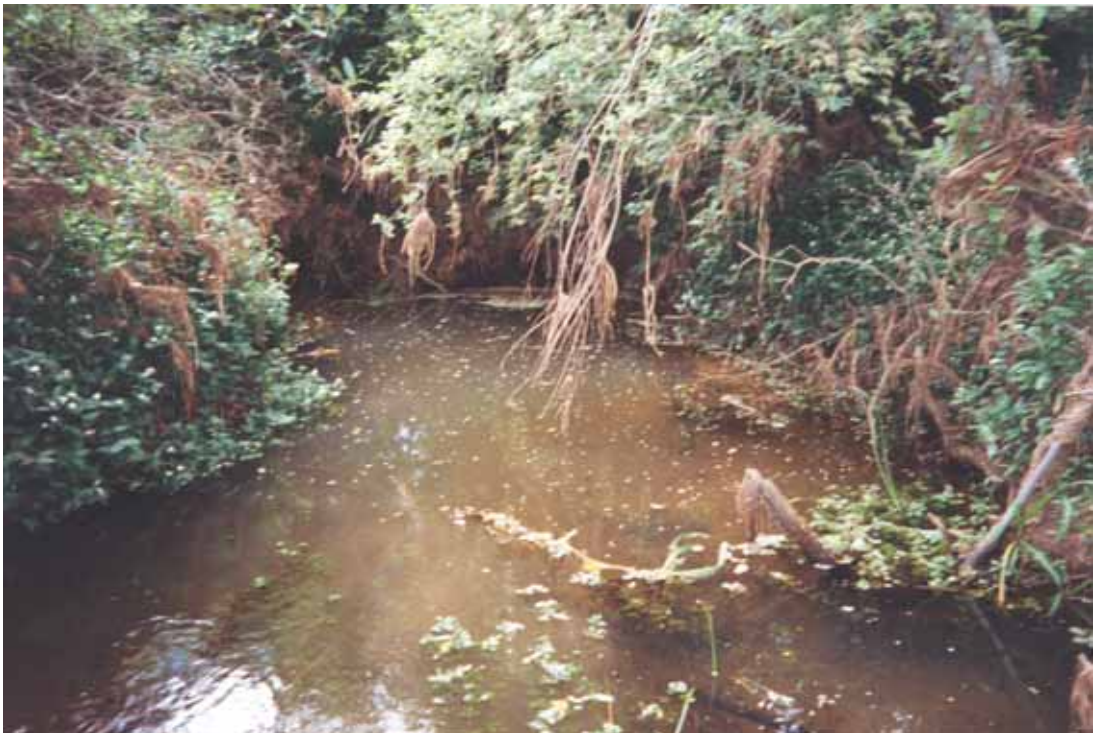
Figure 13.7 A large tree blockage dams the channel at 1.24km above SH2.
