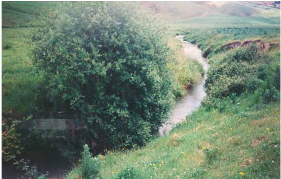
Figure 7.6 Lone tree rooted on the edge of the stream, erosion on a nearby downstream bank.
