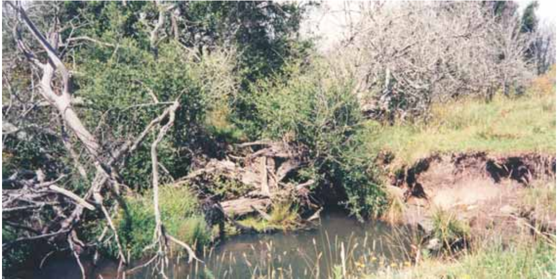
Figure 20.12 Full blockage at 1.1km below SH2.
