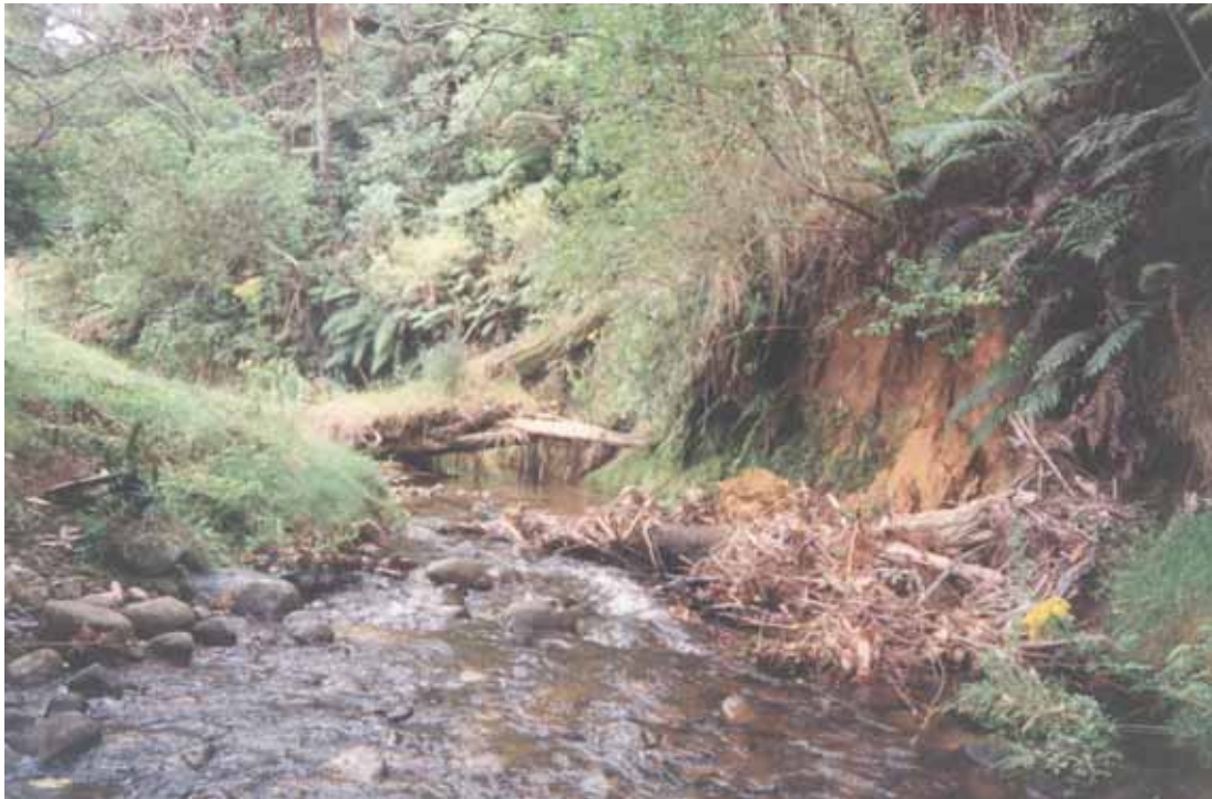
Figure 19.1 Bank erosion at 4.7km. Debris collects on a fallen tree, downstream of this is another partial blockage.
