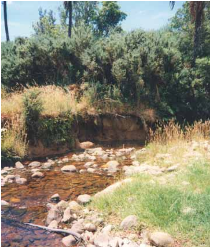
Figure 22.7 The left bank is eroded at 1.2km.
