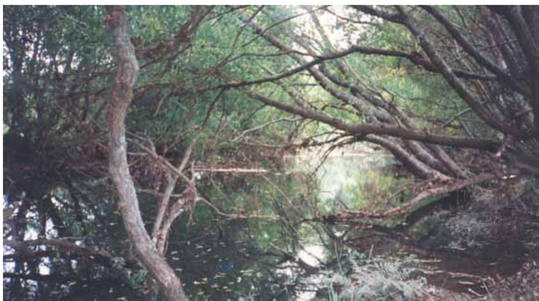
Figure 6.8 Overhanging willows are potential blockages.
