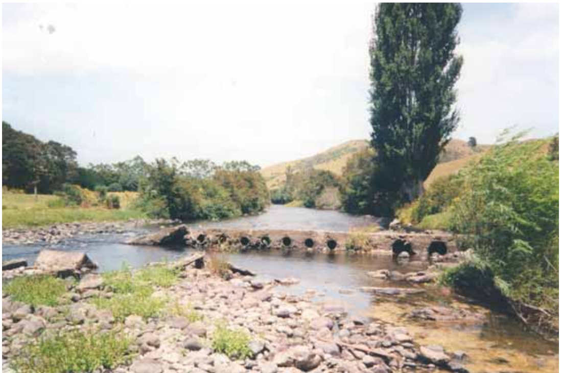
Figure 24.10 At 1.9km a broken causeway lies across the stream..
