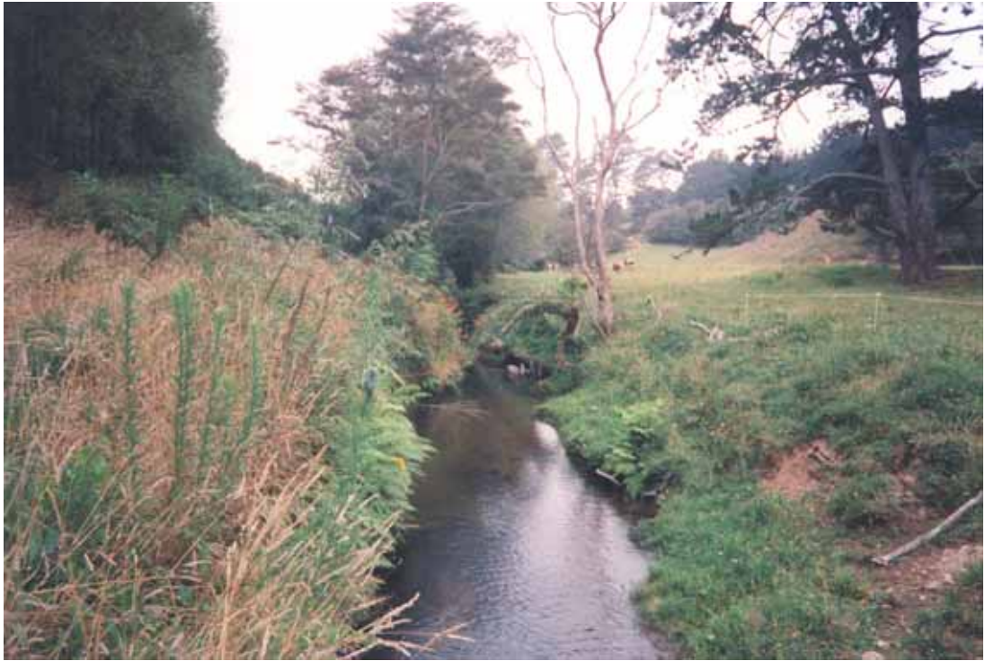
Figure 19.6 Minor erosion of the grassy banks occur at 1.55km.
