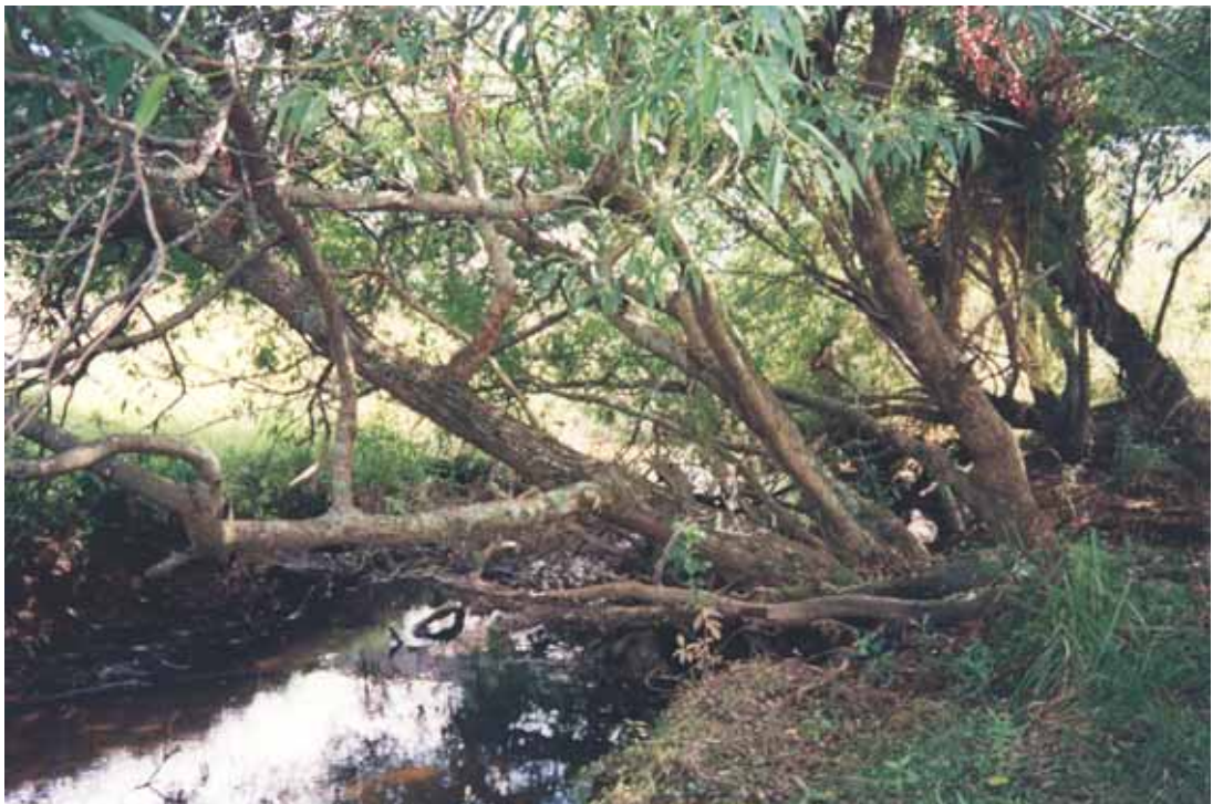
Figure 20.13 Overhanging willows are potential blockages.
