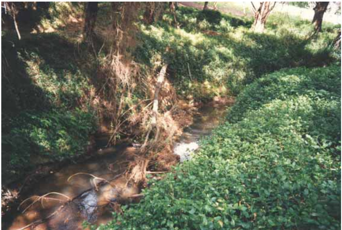
Figure 20.9 Debris collects in the stream and partially blocks the flow. Downstream to the SH2 bridge banks are well vegetated.
