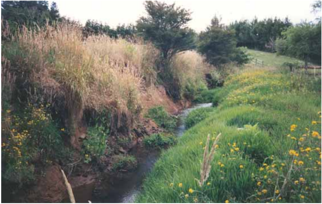
Figure 20.8 Looking upstream at 400m, the true right bank has areas of erosion. The left bank has a good vegetation cover of grass.
