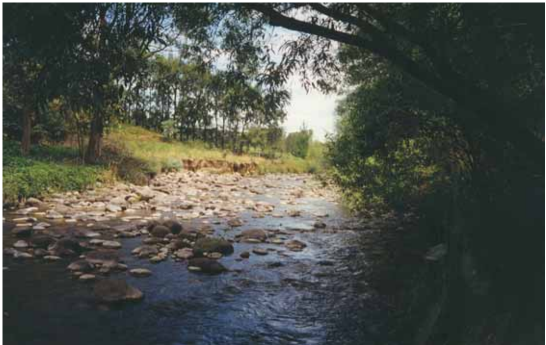
Figure 21.5 Isolated erosion of the true right bank. The bank is vegetated by grasses.
