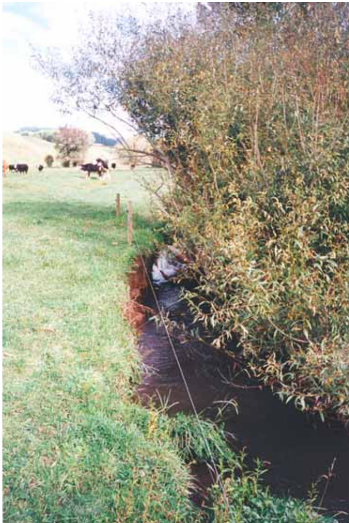
Figure 6.4 Erosion at 2.2km
