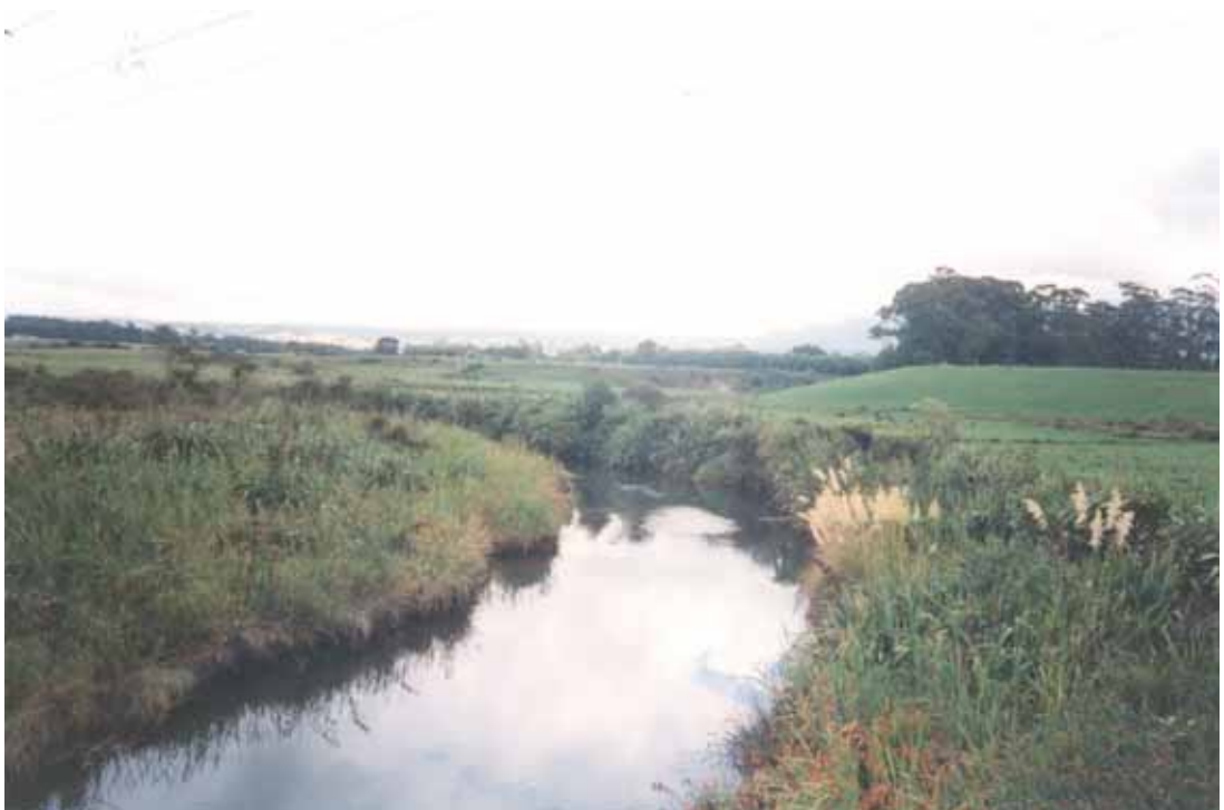
Figure 17.9 For the first 3km above SH2 the banks have good vegetation cover, with little erosion. A wide grassy floodplain extends up to small hills.
