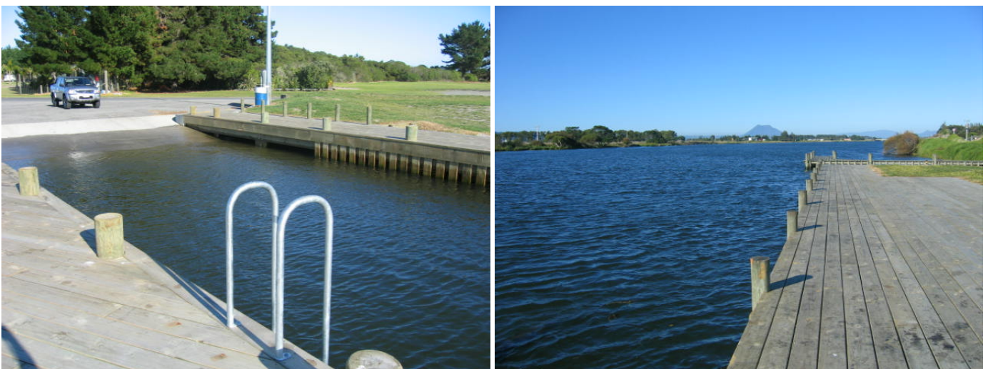
Figure 12: Two views of the launching ramp at Thornton and a view up the Rangitaiki River
