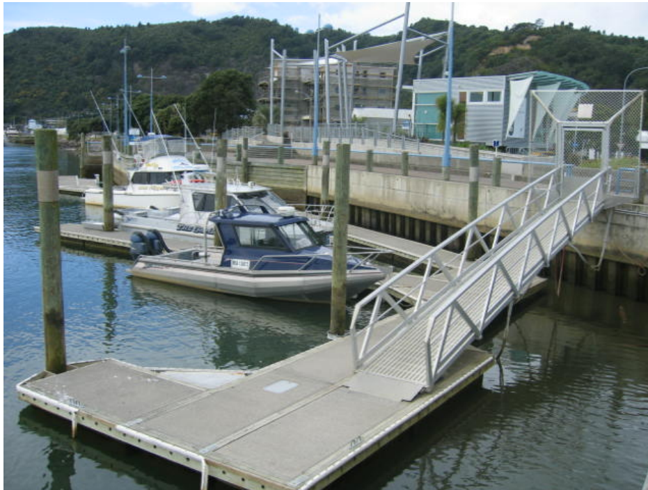
Figure 5: Otuawhaki jetty, whose piles have been extended to prevent it lifting off during a flood event.
