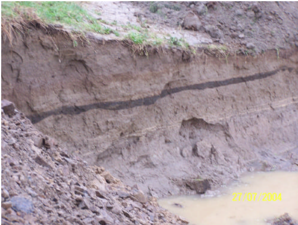
Photograph 6: Exposure at landward toe of stopbank, downstream end of breach showing black Tarawera Ash layer
