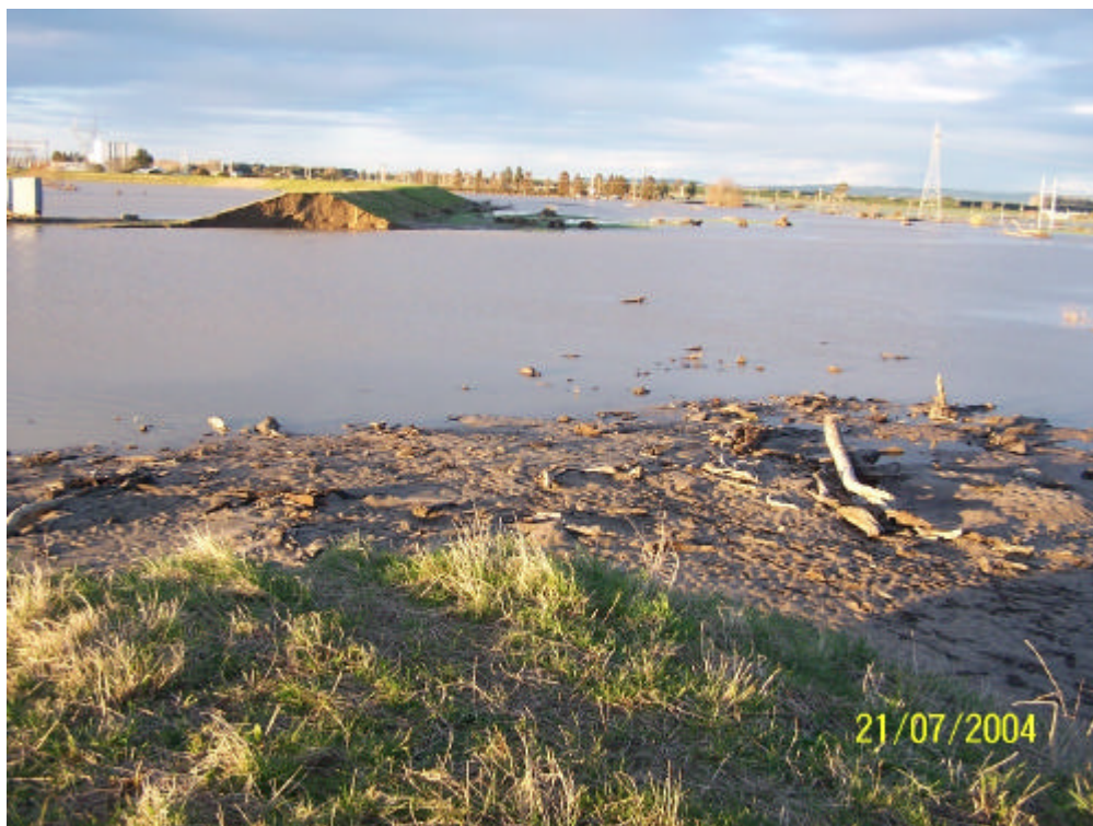
Photograph 2: Looking downstream three days after the initial breach
