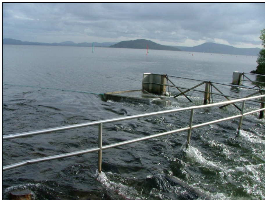
Figure 4: The upstream facing weir trap at the mouth of the Ohau Channel. This trap could only be set when flows were below 20 \text{ m}^3 \text{ s}^{-1} .
