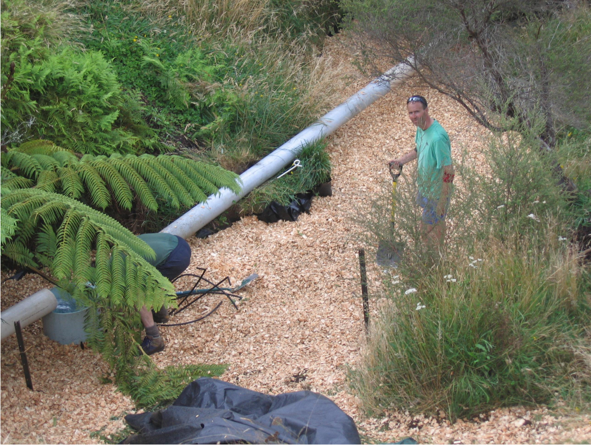
Fig. 1 Bed overview on construction
