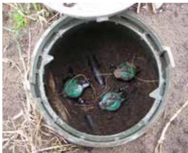
*Where the soak hole option is chosen, the flush valves can be terminated in a chamber over the soakhole*
