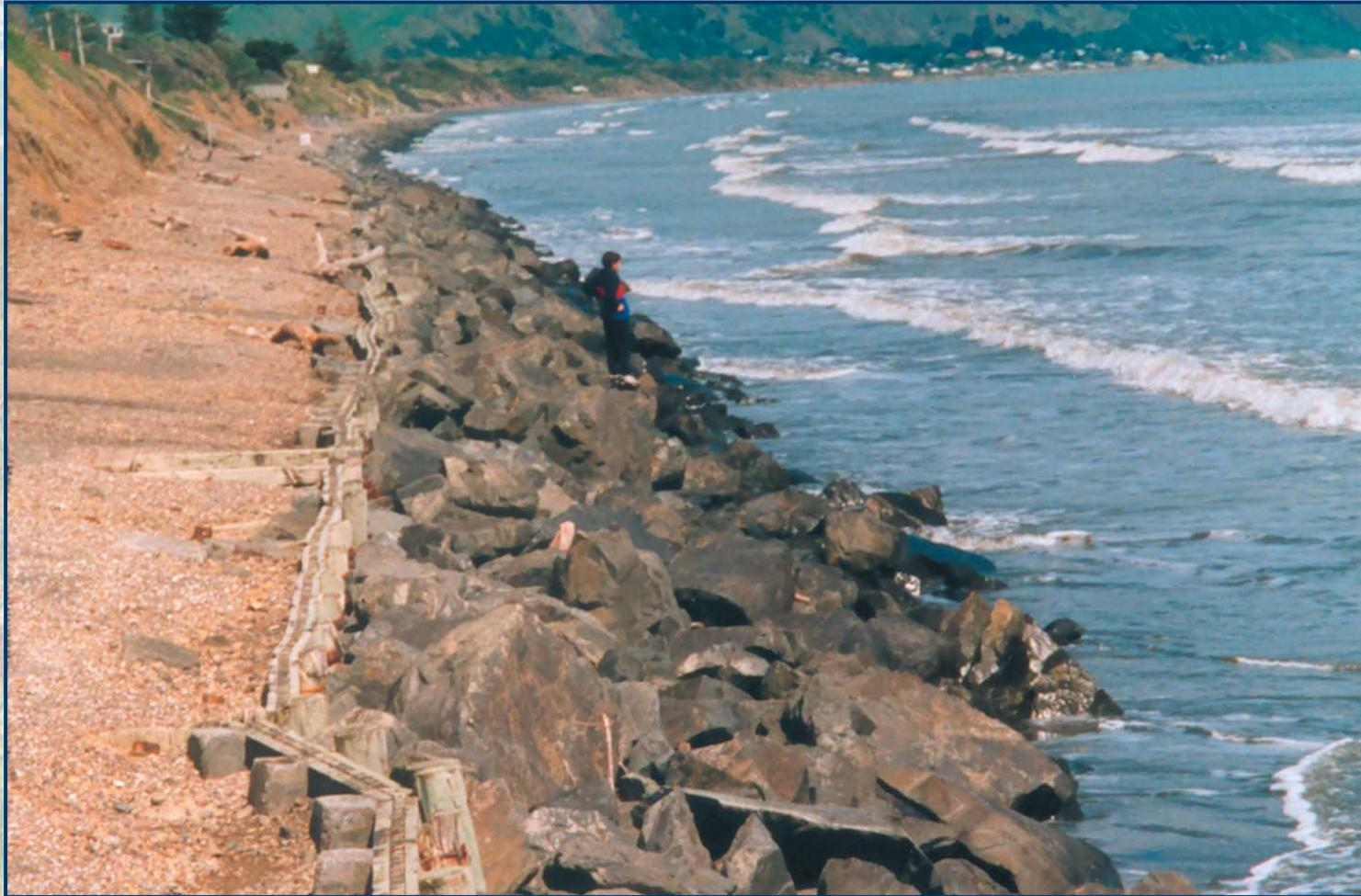
**Rock walls reflect waves and can prevent sand building a safe beach**
