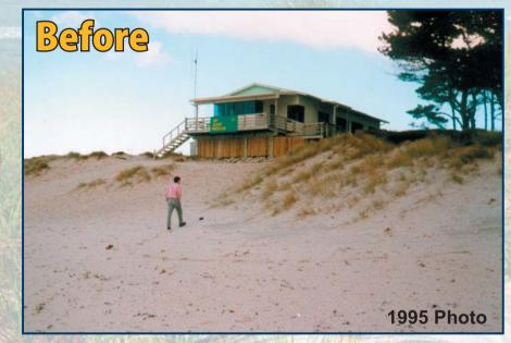
Wind erosion was threatening the stability of the Papamoa Surf Rescue Base (see the broken concrete at the font of the building, placed to reduce wind erosion of the foundations).
