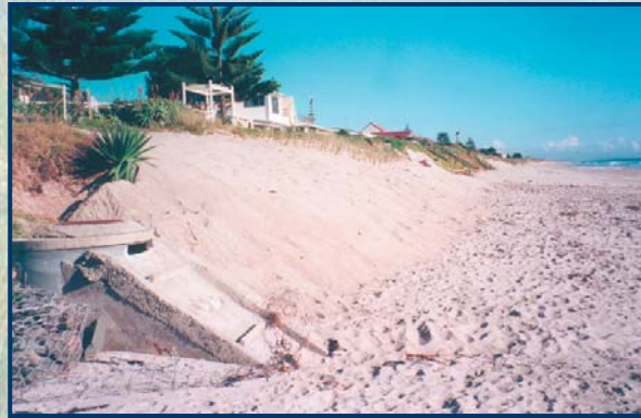
May 2000. During the frequent autumn abundance of sand on beaches, a small quantity was moved up, under strict control by authorities, to reshape the dune front. This sand was planted with spinifex and pingao immediately to stabilise it.
