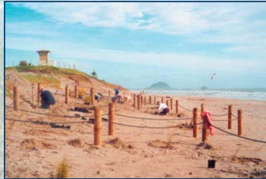
August 2000 Coast Care BOP members desinged, installed and planted leaf shaped plots to create multiple access points. blocking access on occasion.
