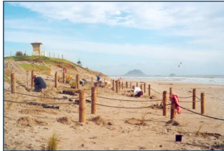
August 2000 Coast Care BOP members designed, installed and planted leaf shaped plots to create multiple access points, blocking access on occasion.
