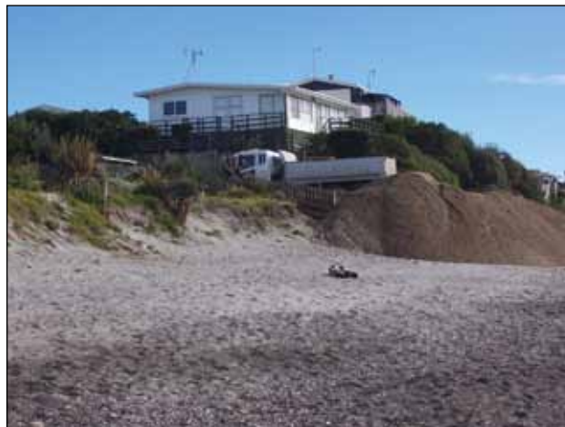
July 2006: Residents paid for sand trucked in from the Pongakawa Canal which was spread in front of their properties.
