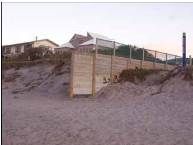
September 2005: 3 weeks after the initial storm damage.
