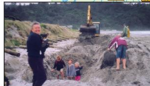
June 2003 All smiles as the removal progresses.
