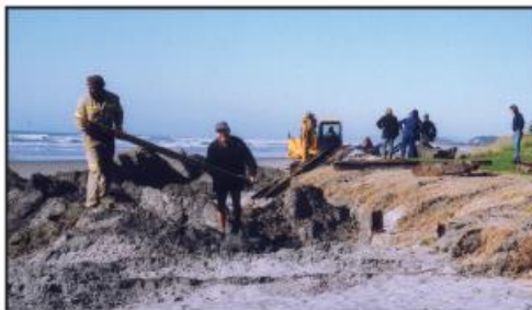
June 2003 First stage of seawall removal with community help.
