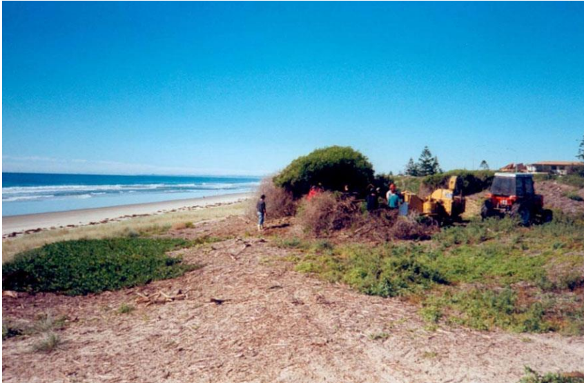
Mount Maunganui wattle clearance 1994
