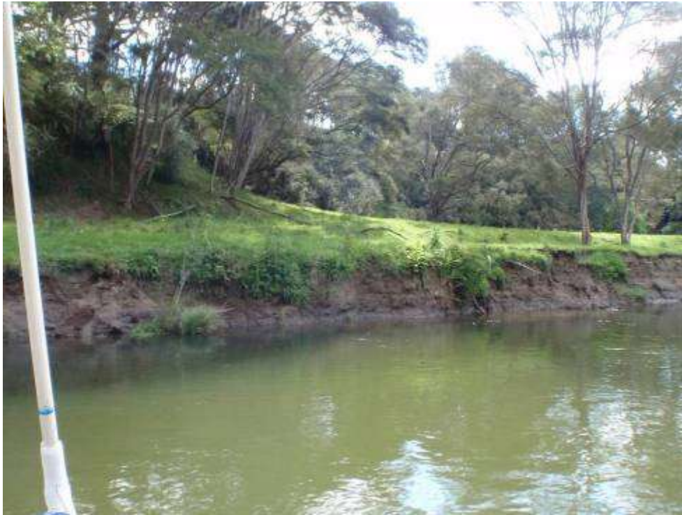
Figure 1-5: Typical 'current scour' type erosion.
