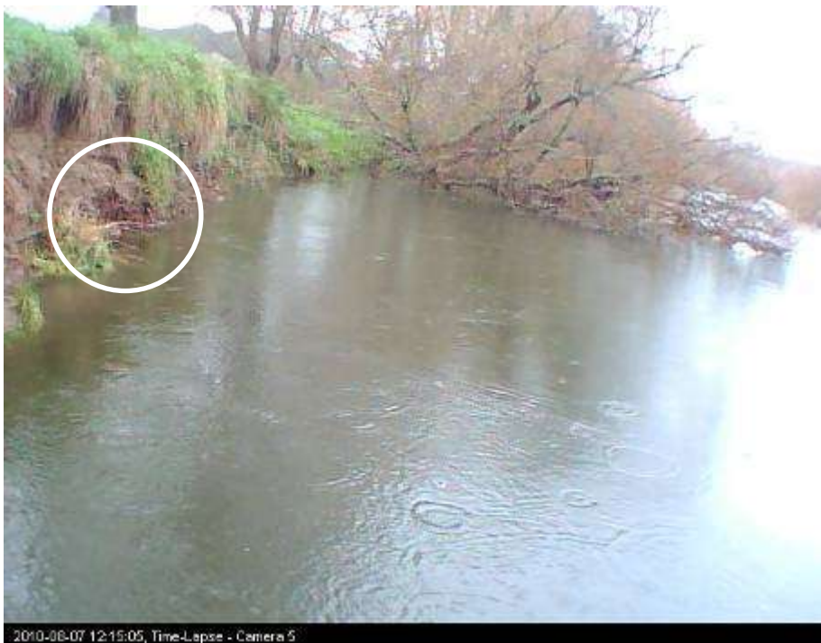
Figure 3-62: Erosion at waters edge of Site 5 on 7/8/10. Compare with previous photo, taken 5 mins earlier.
