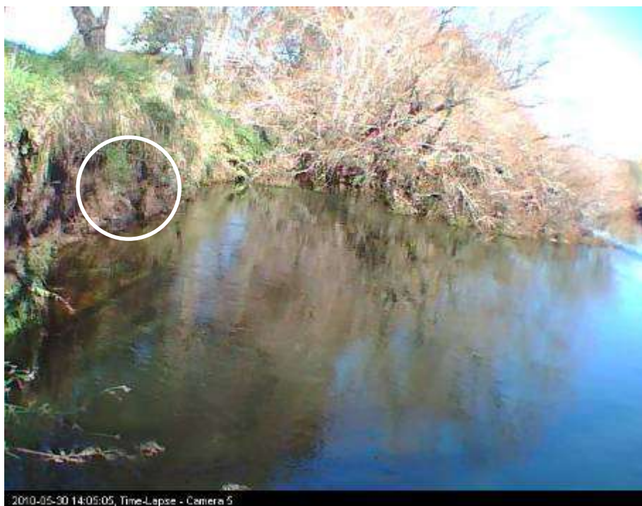
Figure 3-58:Site 5 on the 30/5/10. This is the first clear photo of the bank after floodwaters receded. Note some vegetation removal is circled.
