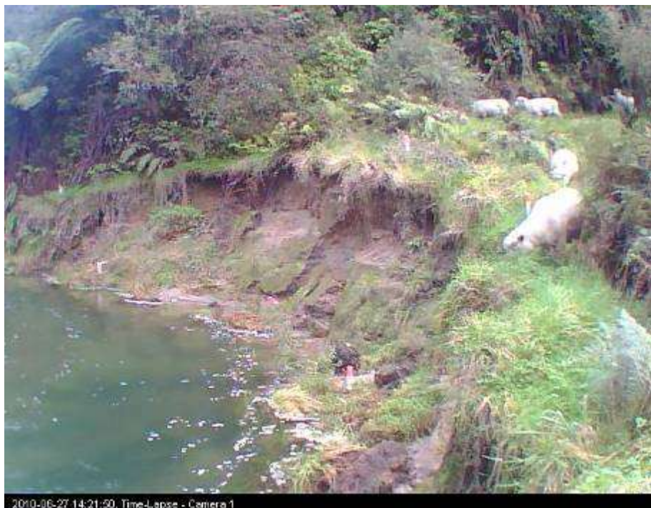
Figure 3-20: Stock access at Site 1 on 27/6/10.
