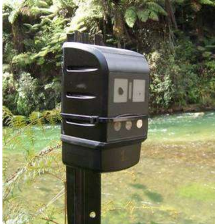
Figure 2-10: The RedEye surveillance camera installed at Site 1.
