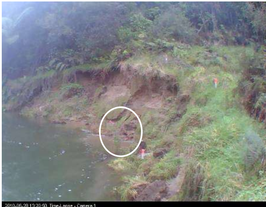
Figure 3-22: Area of erosion at waters edge at Site 1 on 28/6/10. 2 hours after previous photo. Note water discolouration.
