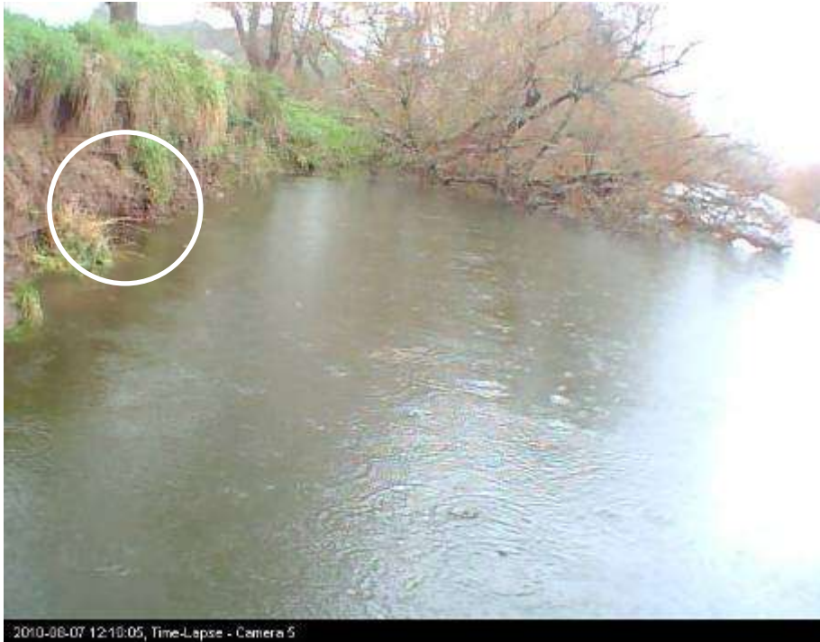
Figure 3-61: Erosion at waters edge of Site 5 on 7/8/10. Compare with following photo.
