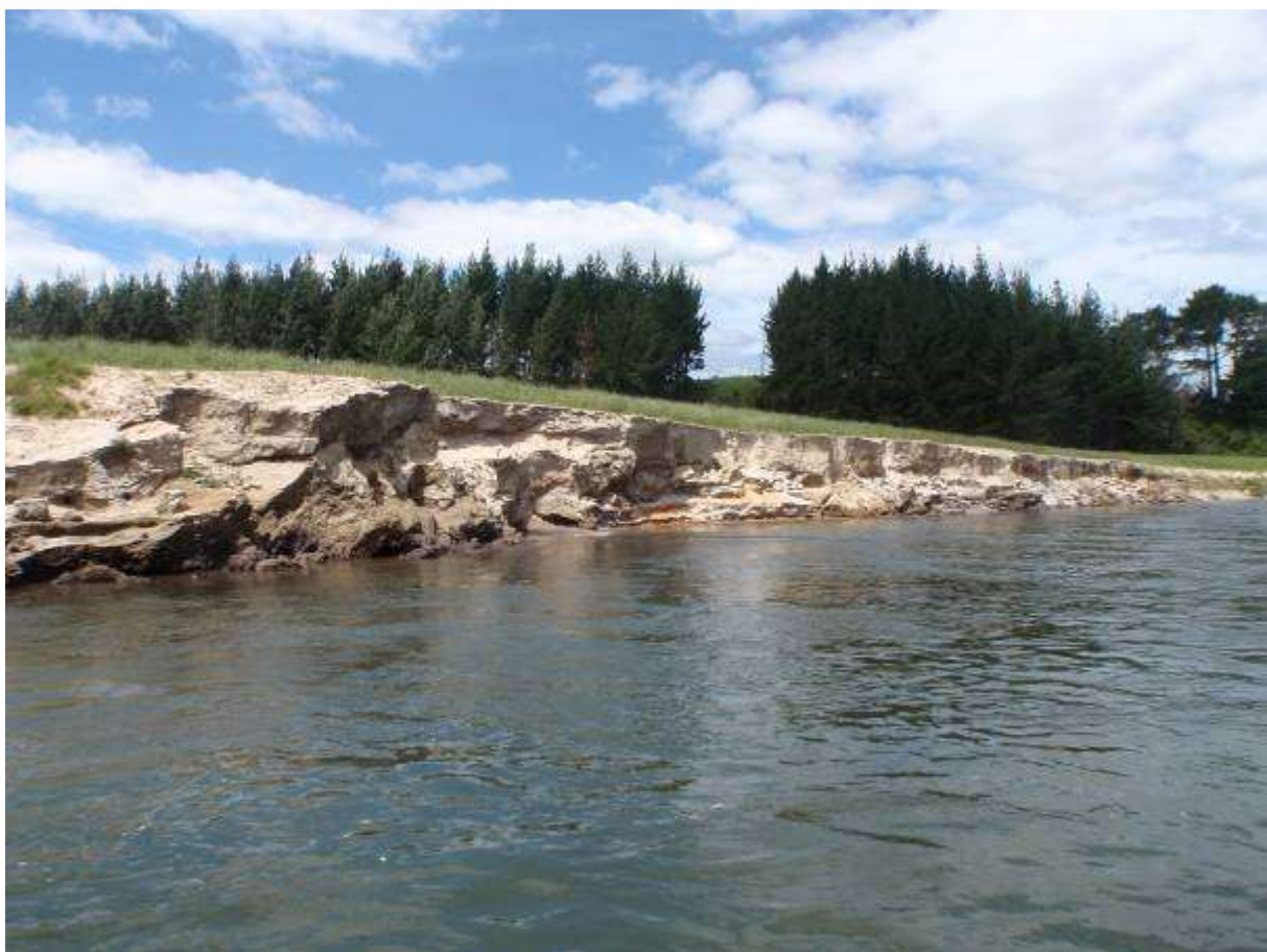
Figure 3-74:Photograph taken at Site 7 on 6/12/10 showing erosion following engineering works.
