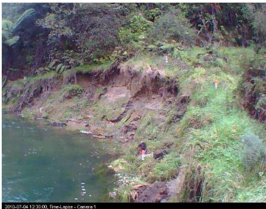
Figure 3-24:Site 1 on 4/7/10 at 12:30. 5 minutes after the previous photo.
