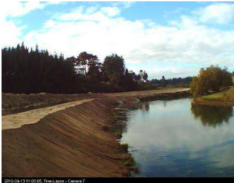
Figure 3-73:Final photograph of Site 7 after engineering works were completed on 13/4/10.
