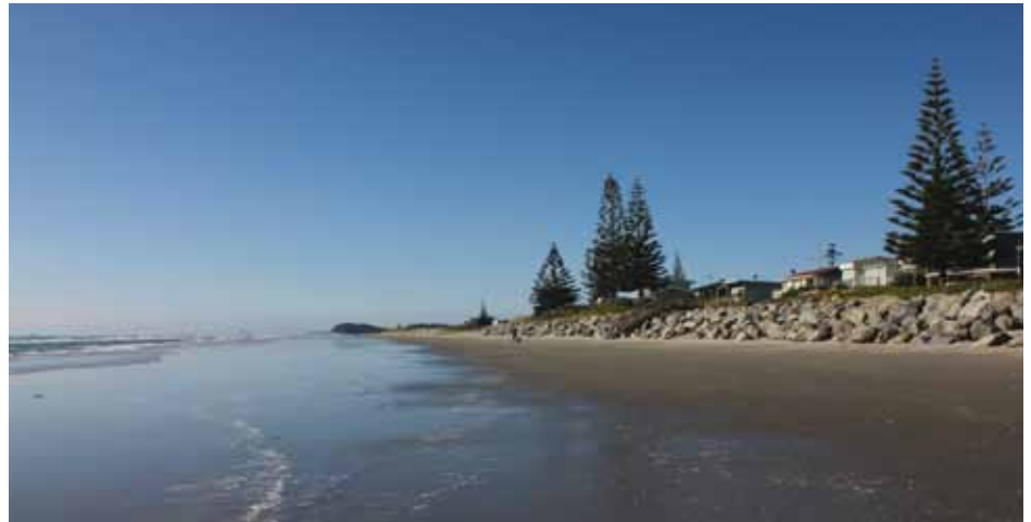
Coastal Protection works, Waihi Beach
