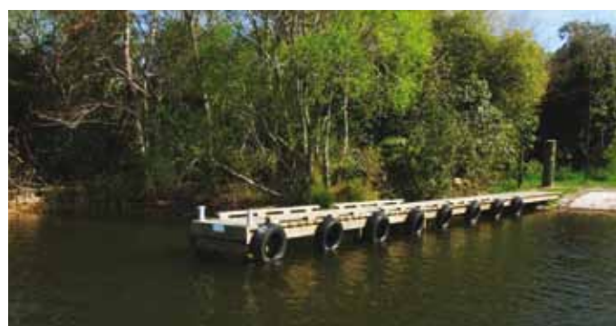
Structures over the bed of the Rotorua Lakes including jetties, platforms, pontoons, retaining walls and ramps will need a resource consent
