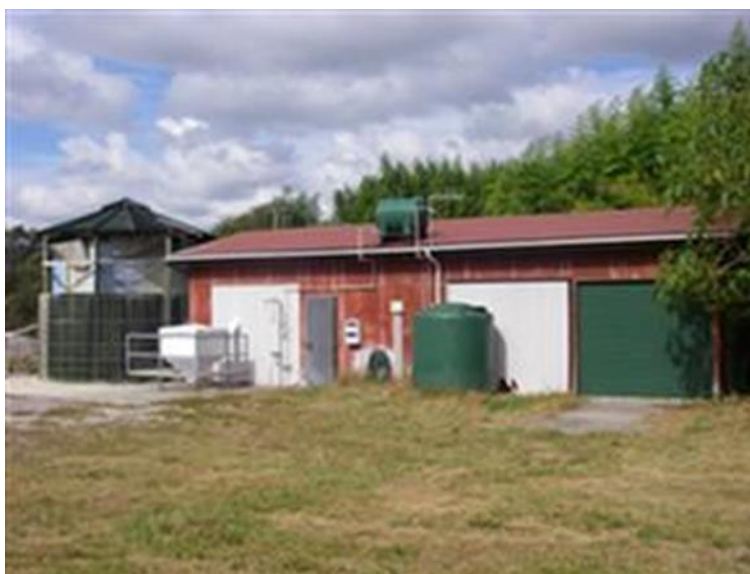
Figure 5 Nitrogen Reduction (De-nitrification) plant.
