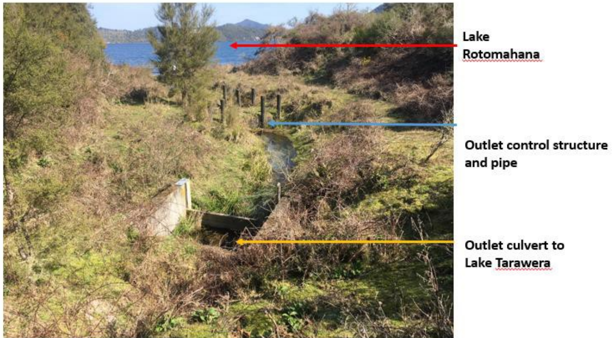
Figure 9 Lake Rotomahana outlet control structure
