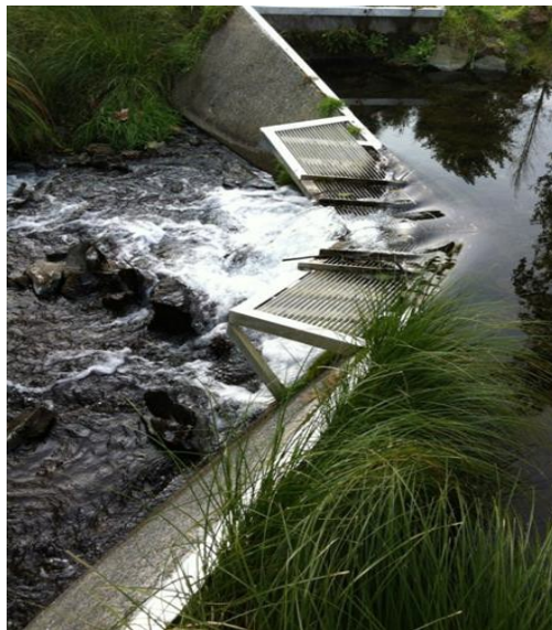
Figure 6 Koaro Fish Pass, Hamurana Stream
