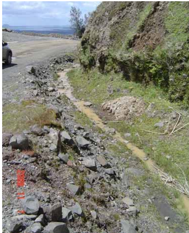
Figure 96 Quarry road access and water table drain leading to control measure – image courtesy of Ridley Dunphy Environmental Limited.
