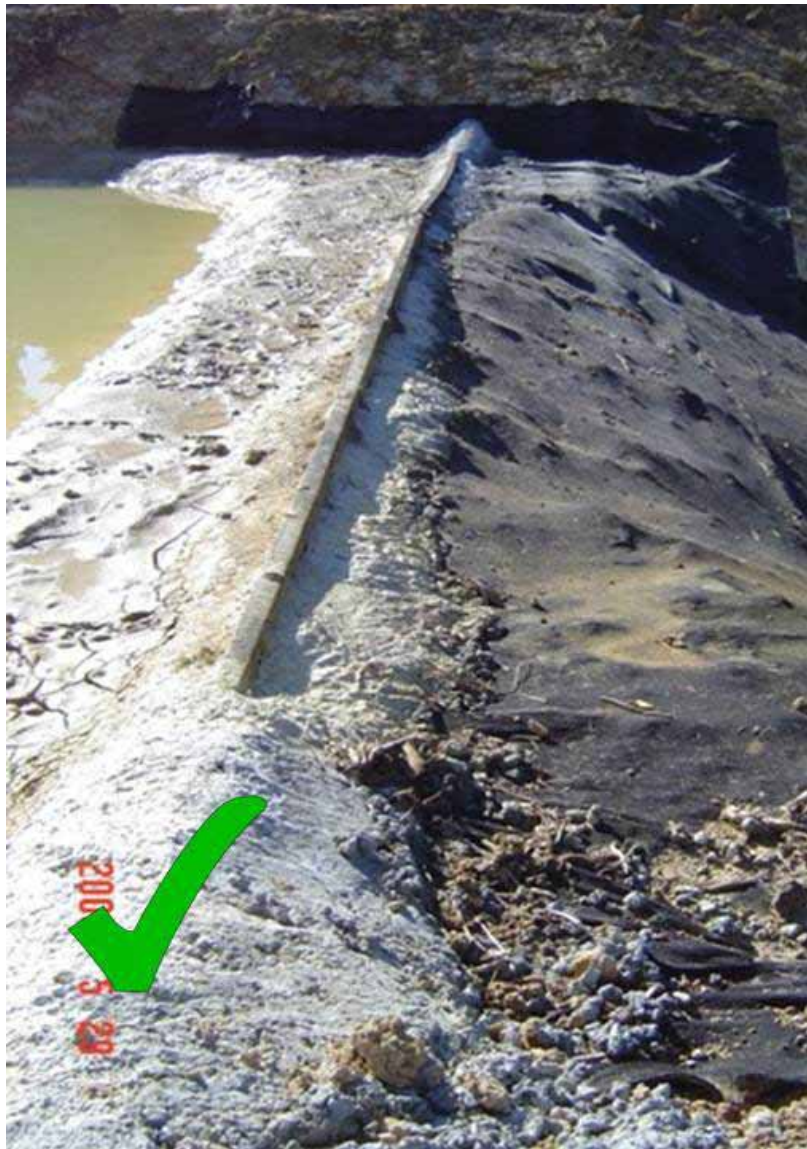
Figure 55 Level spreader showing concrete haunching - courtesy of Ridley Dunphy Environmental Limited.
