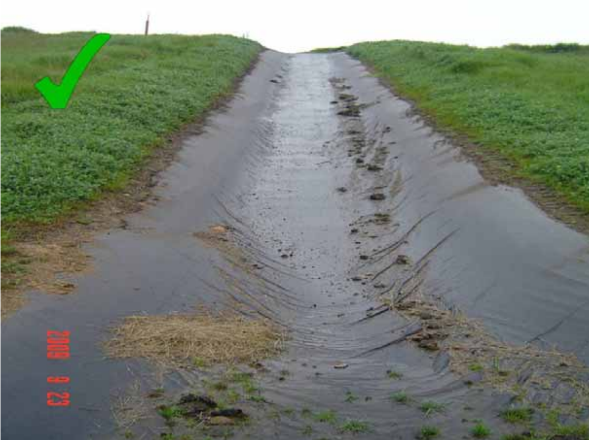
Figure 34 Stabilised flume down a slope - photo courtesy of Ridley Dunphy Environmental Limited.
