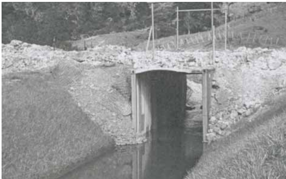
Figure 98 Temporary watercourse crossing – image courtesy of Auckland Regional Council.
