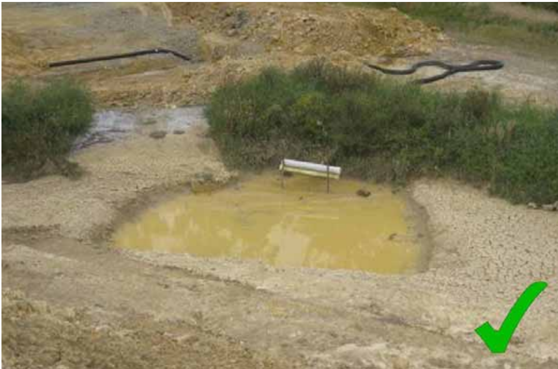
Figure 66 Decanting earth bund installed with "T"-bar decant.
