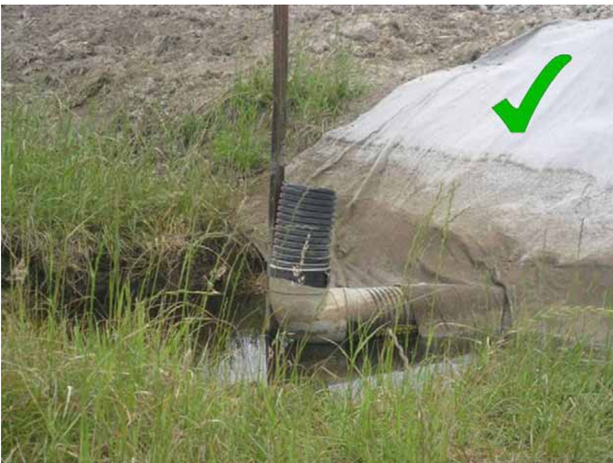
Figure 69 Snorkel upstand decant.
