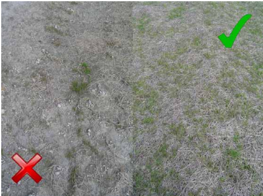
Figure 16 Good and inadequate mulch surface cover - photo courtesy of Ridley Dunphy Environmental Limited.
