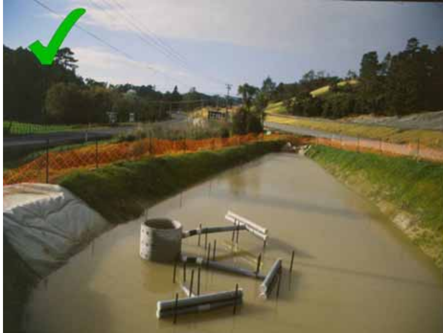
Figure 52 Sediment retention pond - photo courtesy of Auckland Regional Council.
