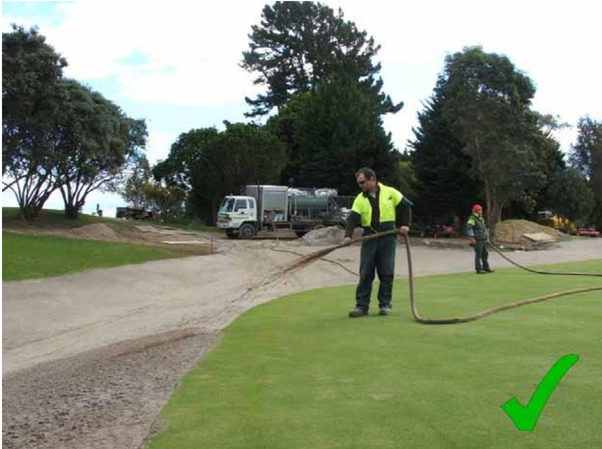
Figure 10 Hydro seeding Operation - photo courtesy of Erosion Control Limited.
