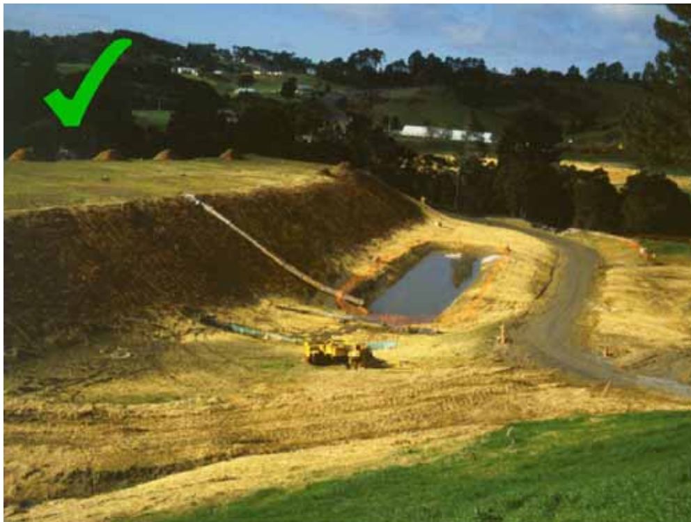
Figure 37 Flume discharging to appropriate sediment retention pond with no slope scour. Photo courtesy of Auckland Regional Council.
