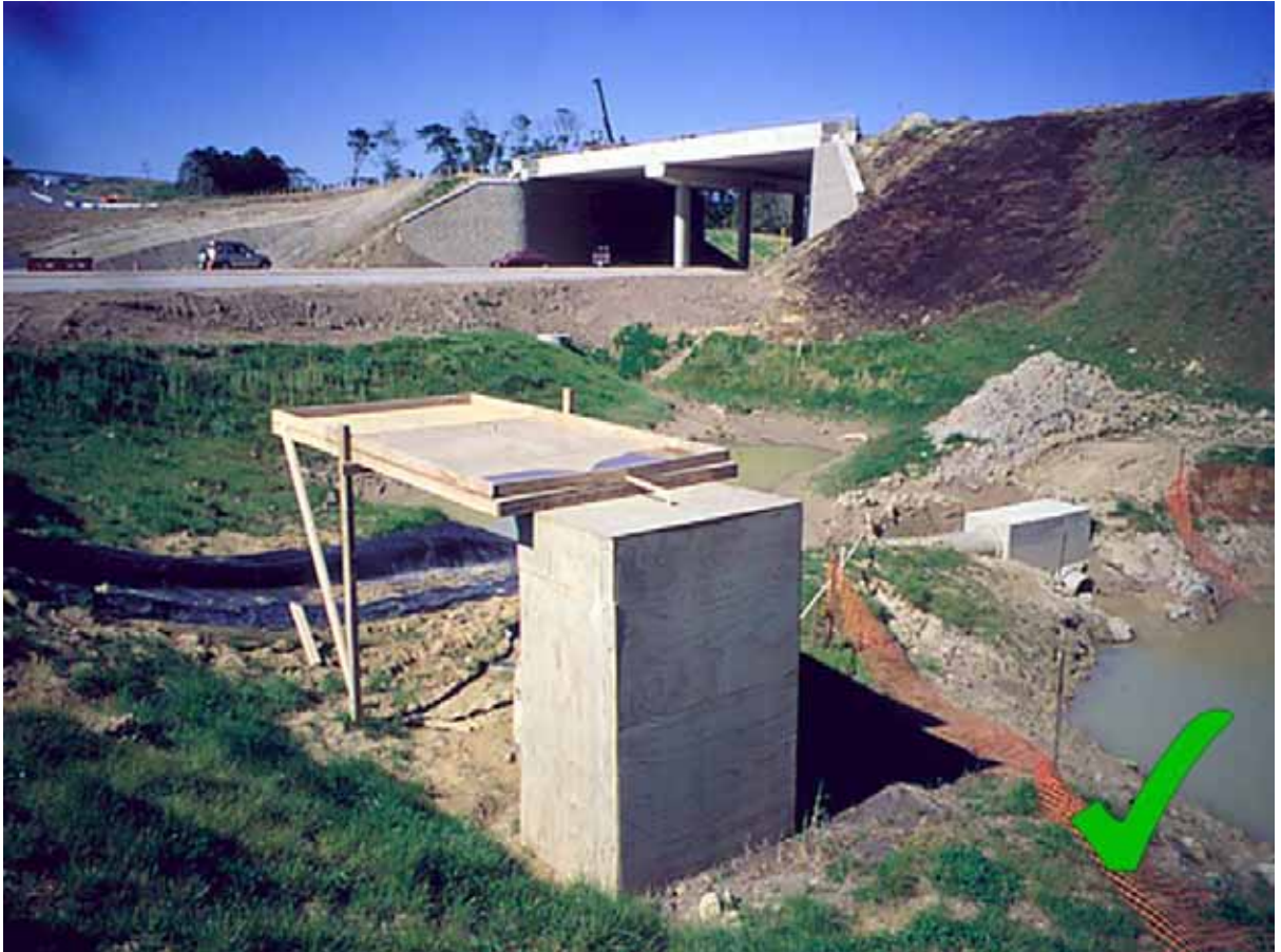
Figure 92 Operation chemical treatment system – image courtesy of Auckland Regional Council.
