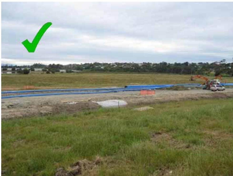
Figure 67 Decanting earth bund installed along the contour.
