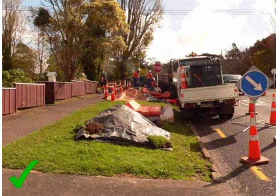
Figure 20 Geotextile covering of stockpiles - photo courtesy of Site Specific Limited.
