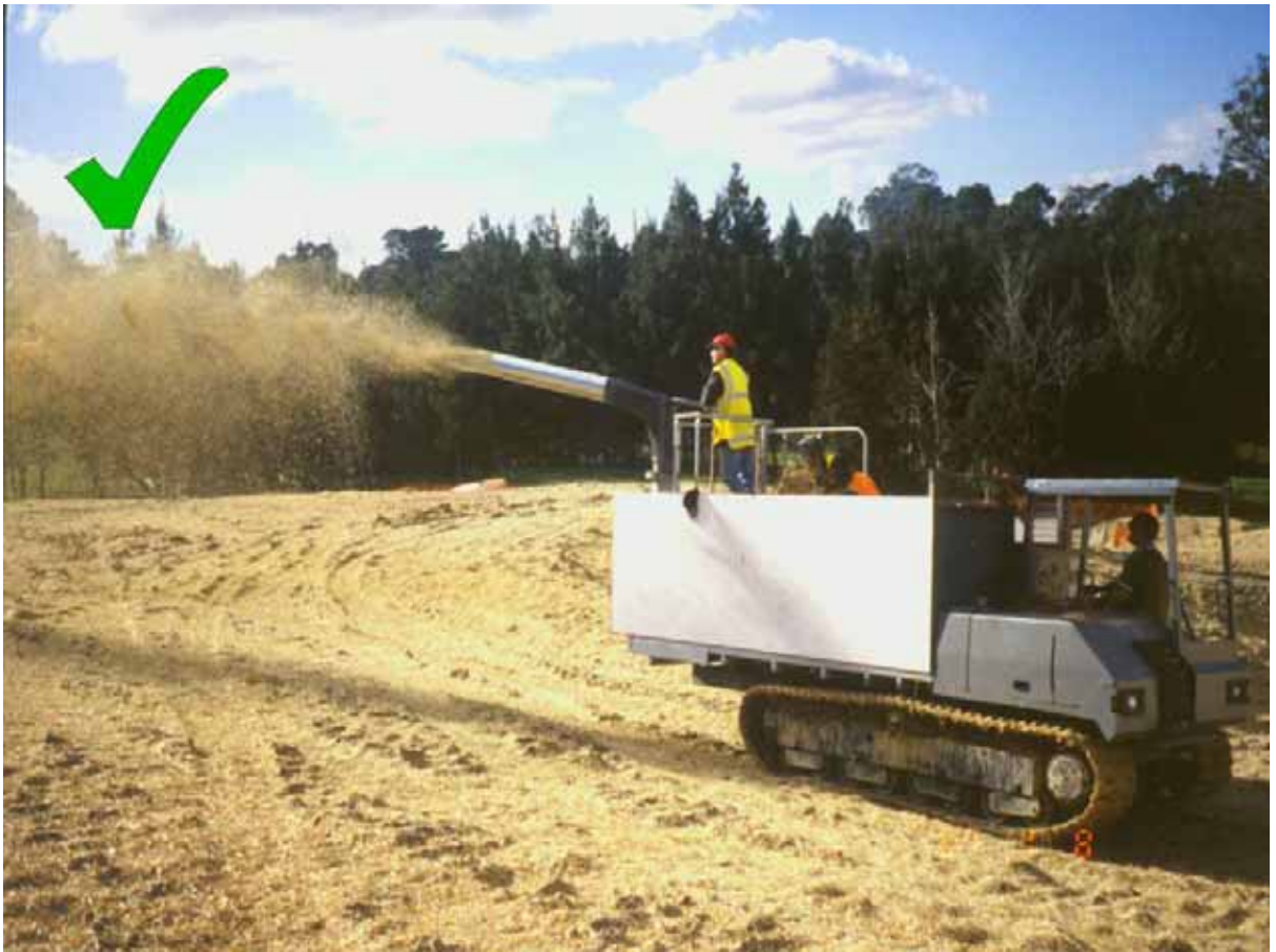
Figure 13 Specialist application of hay mulch - photo courtesy of Auckland Regional Council.
