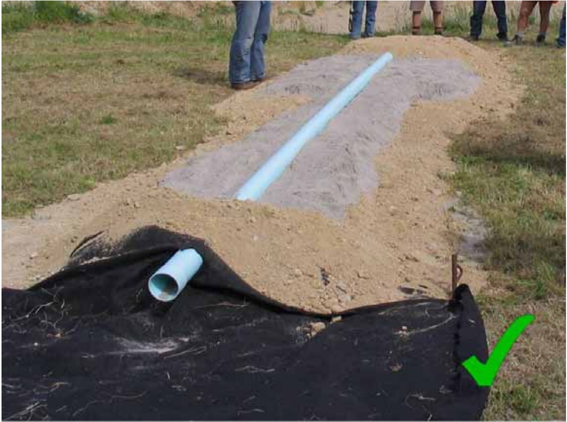
Figure 57 Approved antiseep collar design - Courtesy of Wai Ora Soil Conservation Limited.
