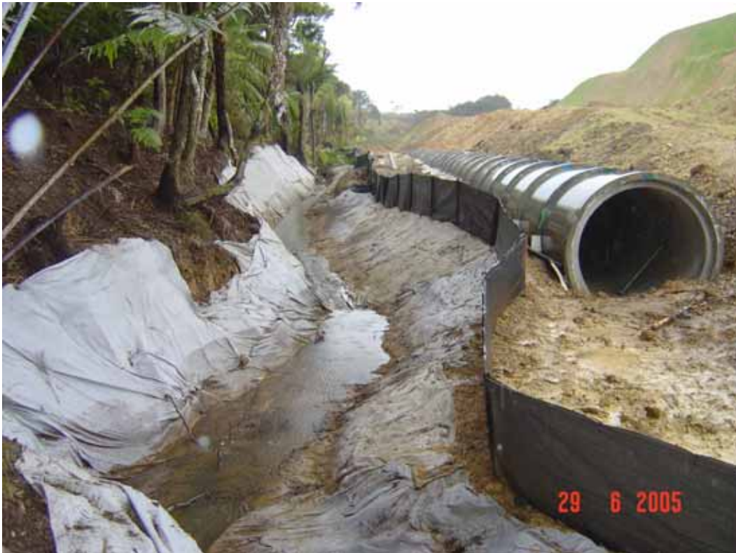
Figure 99 Temporary watercourse diversion – image courtesy of Auckland Regional Council.
