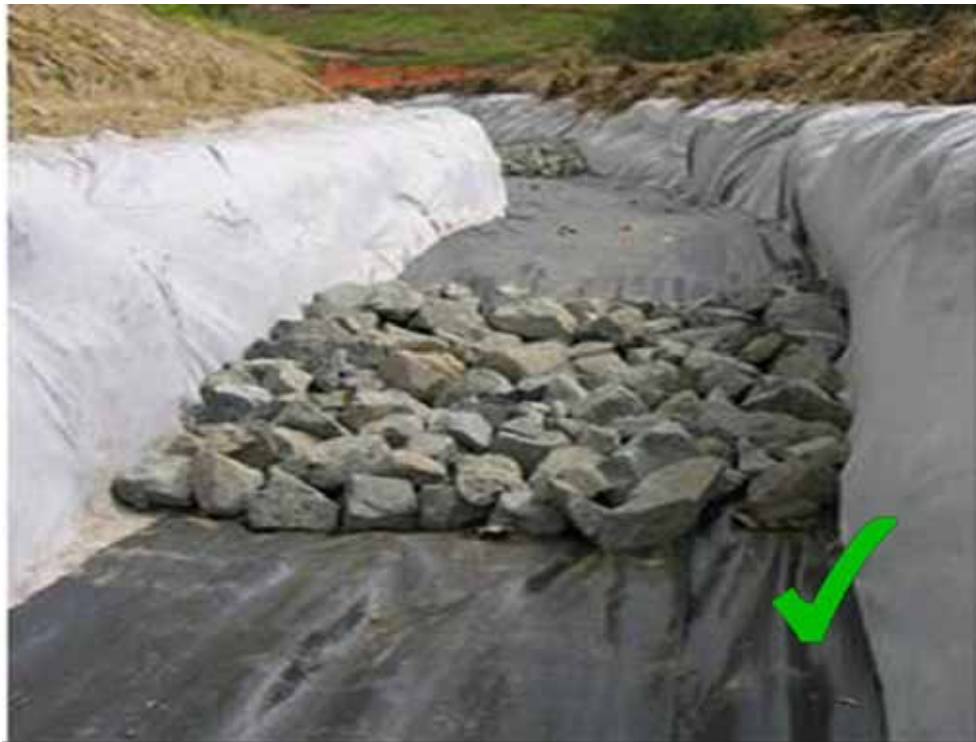
Figure 40 Check dam using rock rip rap. Good spacing of check dams and fabric lining of channel however rock should be shaped to provide a spillway - photo courtesy of Environment Canterbury.
