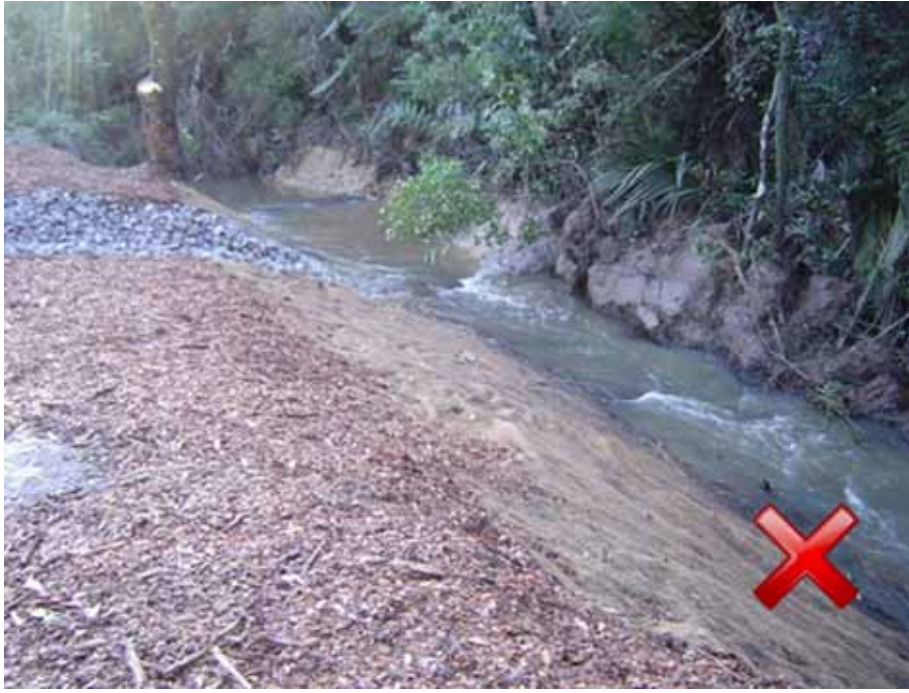
Figure 22 Geotextile with fine mesh on stream bank causing potential damage to wildlife through trapping in mesh system – photo courtesy of Ridley Dunphy Environmental Limited.
