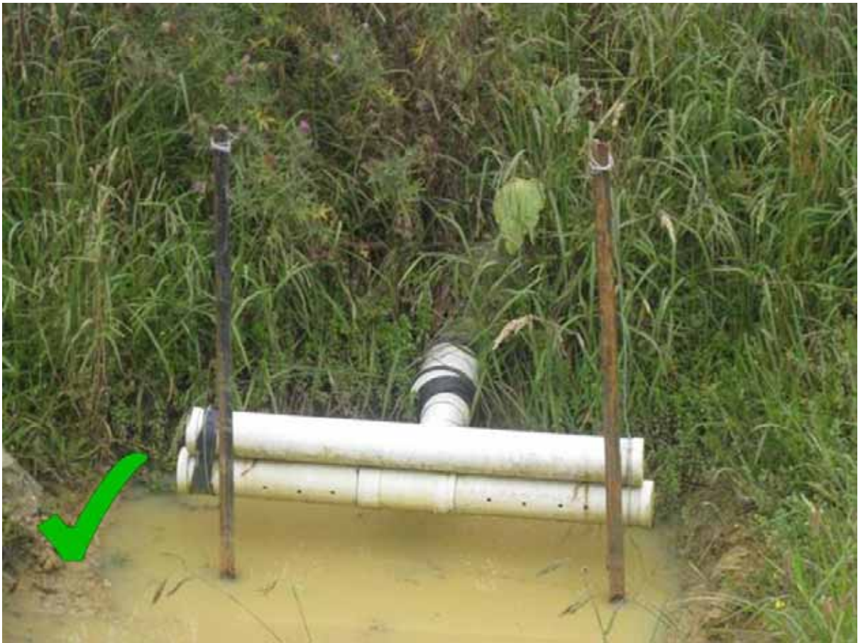
Figure 68 T-bar decant.
