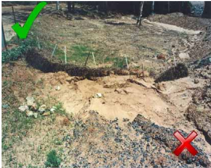
Figure 85 Hay bale barrier – Good use of stakes however in concentrated flow path - photo courtesy of Auckland Regional Council.
