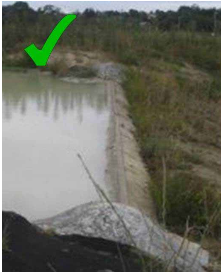
Figure 49 Level spreader construction - photo courtesy of Ridley Dunphy Environmental Limited.
