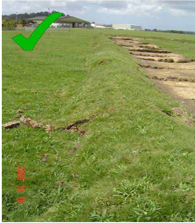
Figure 30 Example of stabilised clean water diversion channel – stabilised with grass sward. Photo courtesy of Ridley Dunphy Environmental Limited.
