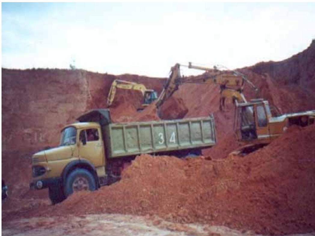
Figure 97 Quarry overburden removal – image courtesy of Google images.
